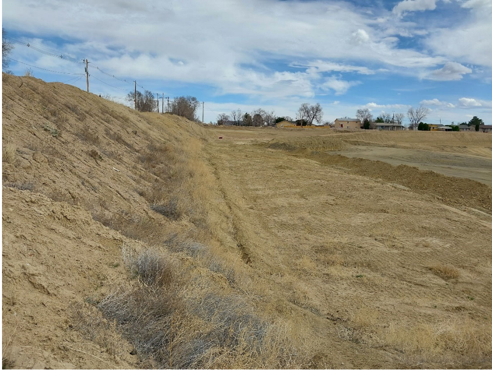
Photo #19: South side of berm along the north side of permit boundary and affected area, looking east. Slope is at an angle of repose but appears to be stable.
