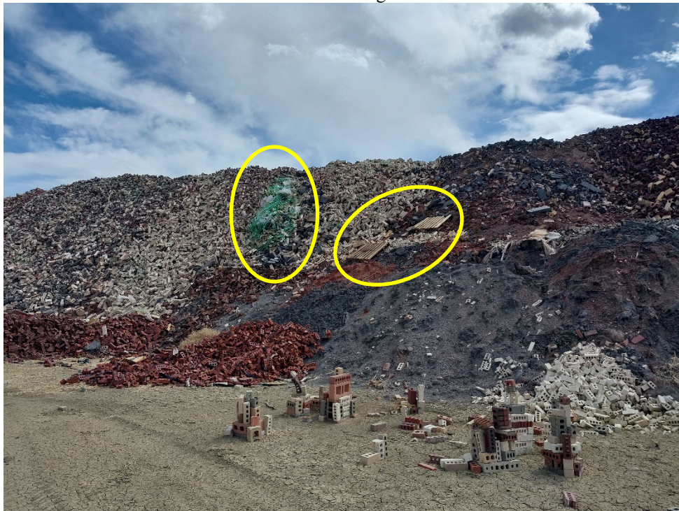
Photo #24: Plastic banding and wooden pallets seen in the discarded brick stockpile to be used for backfilling material. Operator needs to remove these items as they are not inert and cannot be used as backfilling material.
