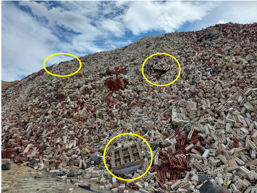
Photo #25: Plastic banding and wooden pallets in the discarded brick stockpile to be used as backfilling material. Operator needs to remove these items as they are not inert and cannot be used as backfilling material.
