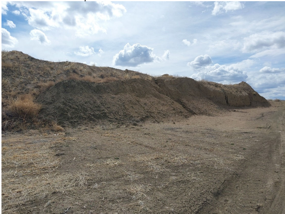
Photo #28: North side of topsoil stockpile, looking west southwest. This slope is at an angle of repose, is not vegetated, and is not stable. There are incisions in the material that can be viewed. Operator needs to repair this slope and restabilize the topsoil stockpile.
