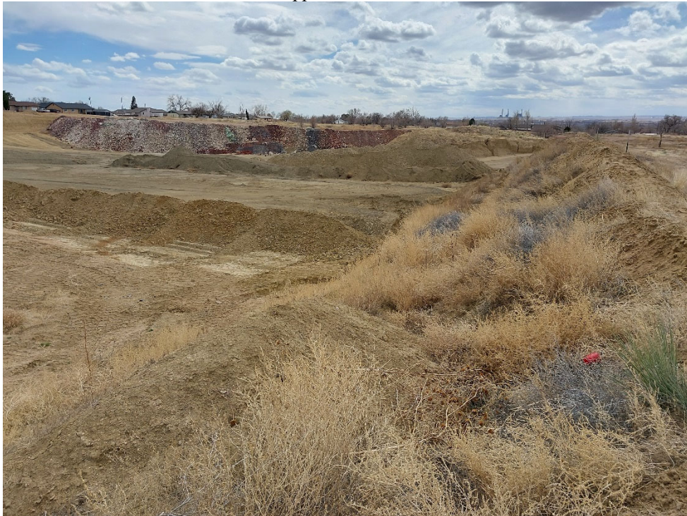
Photo #20: The right side of the photo shows the north-south berm around the affected area, looking south. Slopes are at angle of repose but appear to be stable. The discarded brick stockpile, topsoil stockpile, and product stockpile can be seen in the background in the center and left of the photo.
