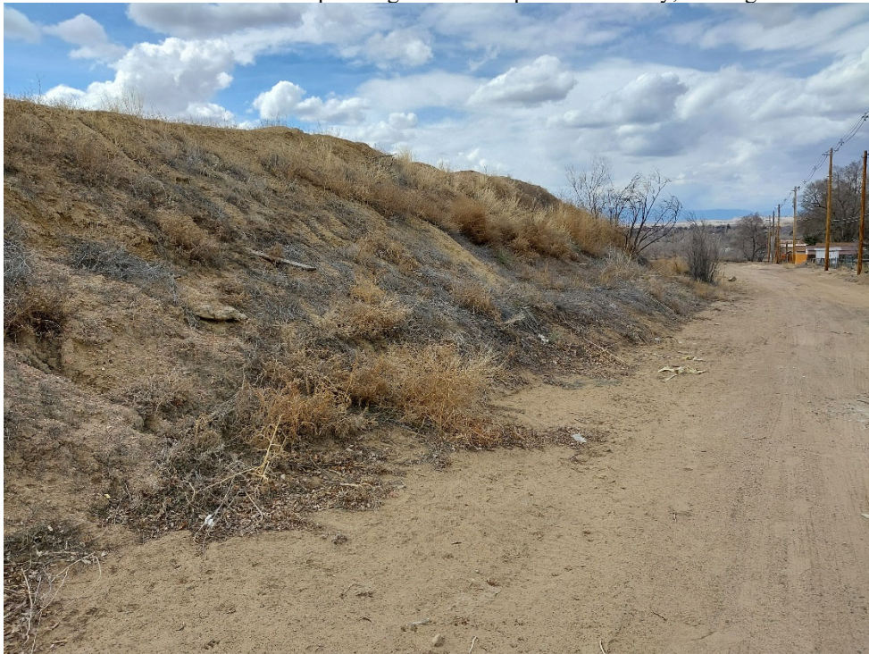
Photo #18: North side of berm along the north side of the permit boundary, looking west. Slope is at angle of repose but is well vegetated and appears to be stable.
