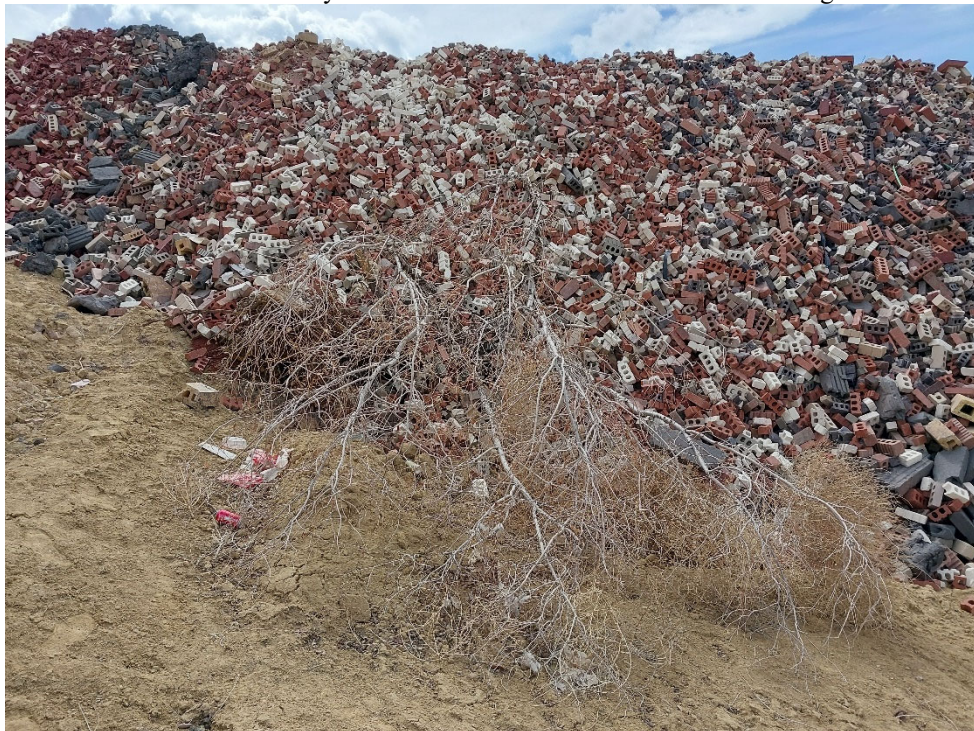
Photo #26: Tree that has been buried by discarded brick dumping. Operator needs to remove item it is are not inert and cannot be used as backfilling material.
