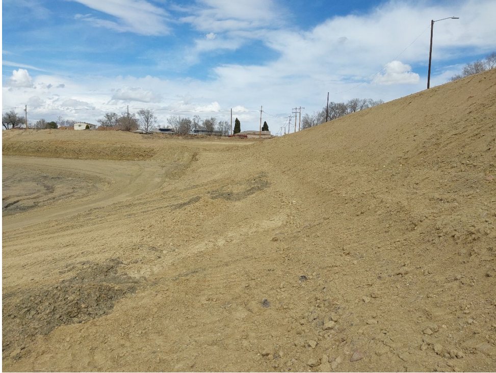
Photo # 17: Graded 3:1 slope along the eastern permit boundary, looking north.
