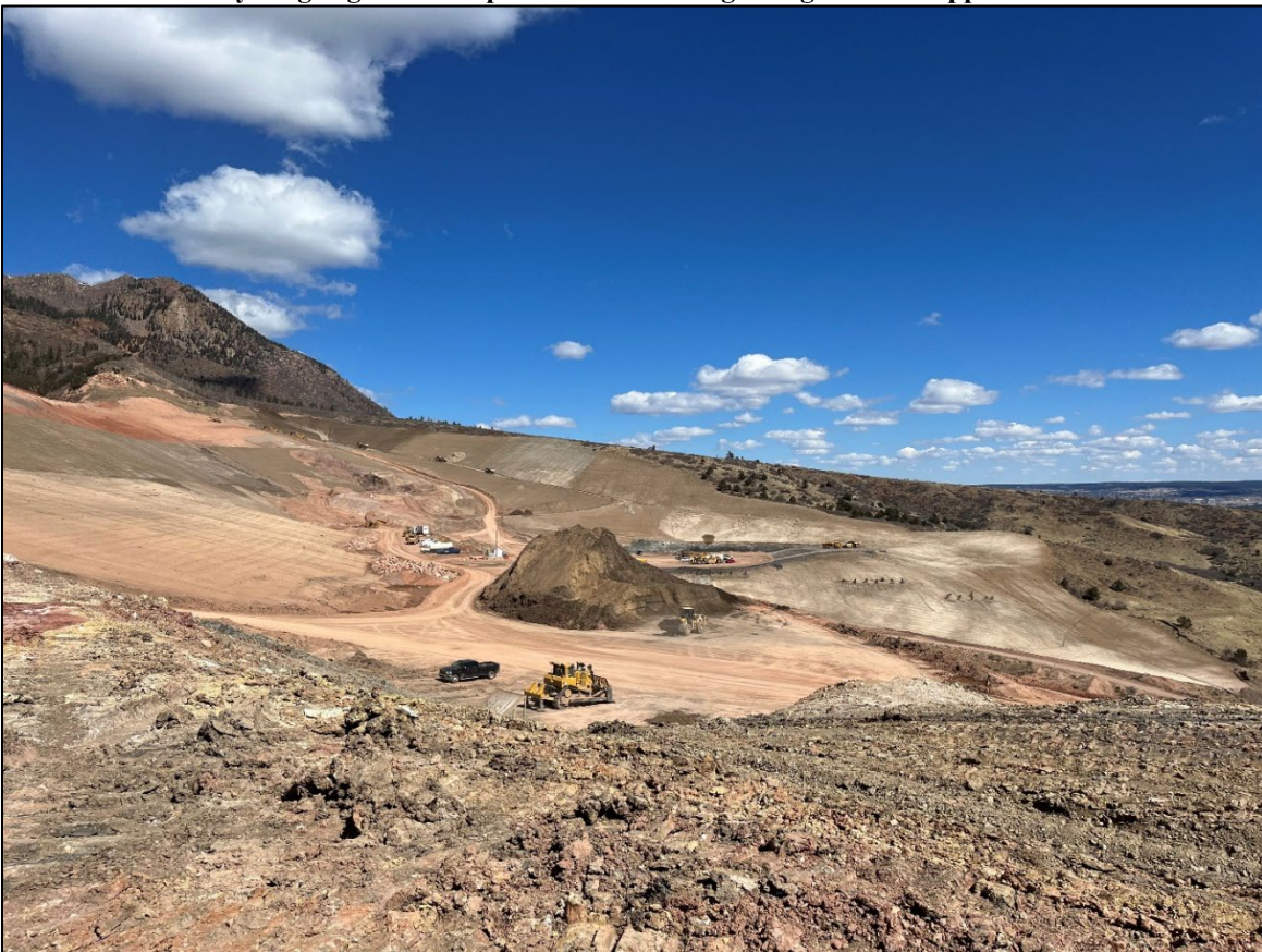
Photo 4: View north from the south borrow area, a topsoil pile is located in the foreground. The revegetated northern slope is visible in the foreground.
