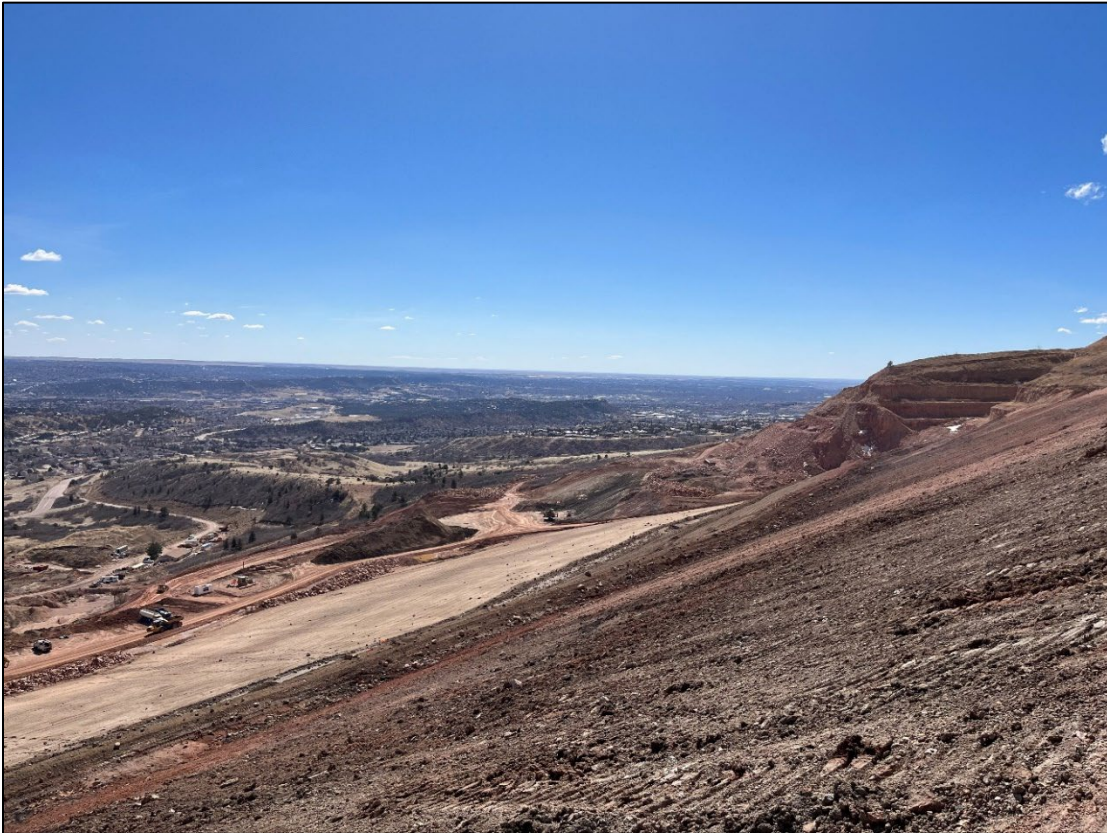
Photo 1: View SE of the lower and south borrow areas, taken from level 4.
