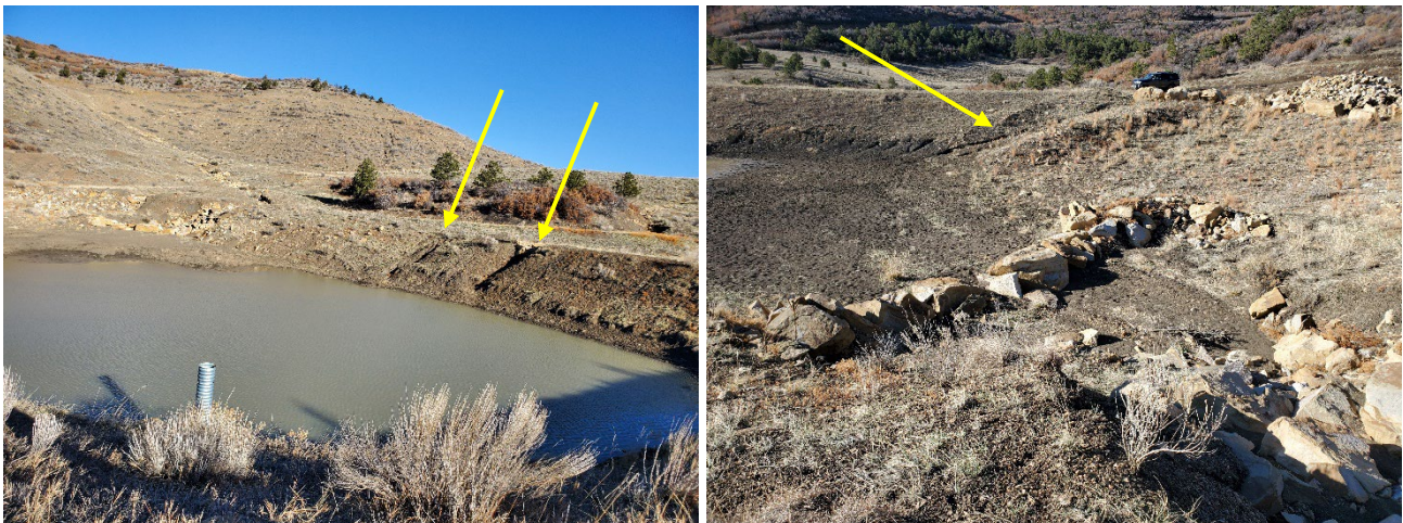
Photo 2: Pond 006a. Arrows indicate the erosion on the north (left photo) and west (right photo) banks.
