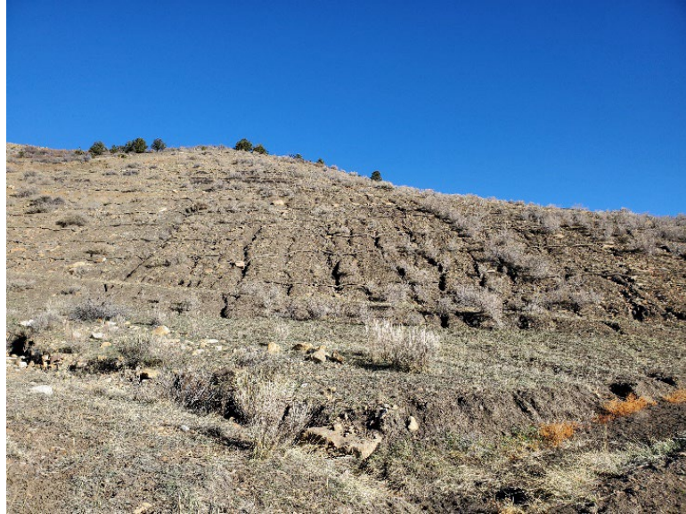
Photo 8: Erosion on the reclaimed area above and west of Pond 006a.
