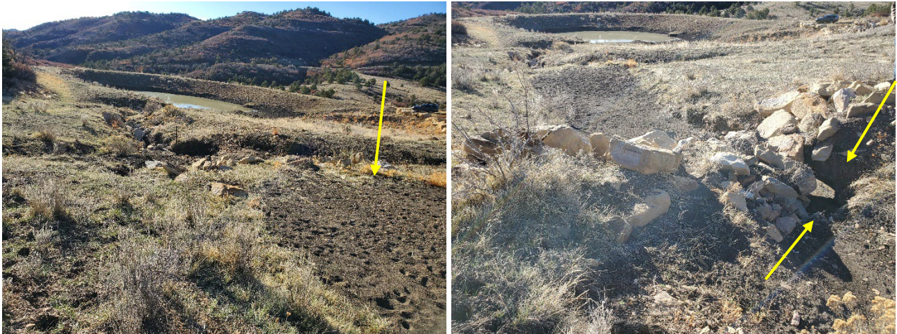
Photo 6: (Left) Arrow points to a check dam that is nearly full of sediment (see Maintenance Item #3a). (Right) Arrows point to an area where water has undercut a check dam along its southern bank (see Maintenance Item #3a).
