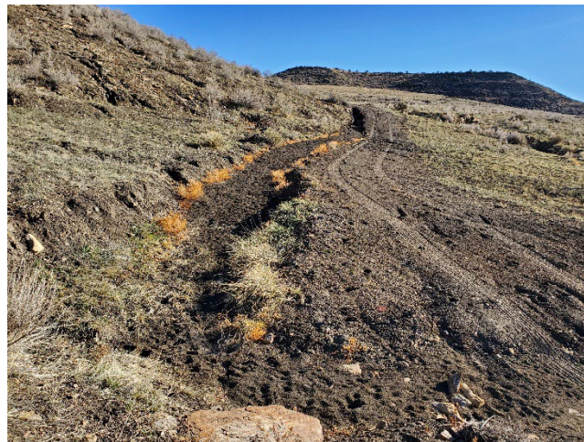
Photo 7: Ditch along the west side of the access road to Pond 006a that is full of sediment (see Maintenance Item #3b).
