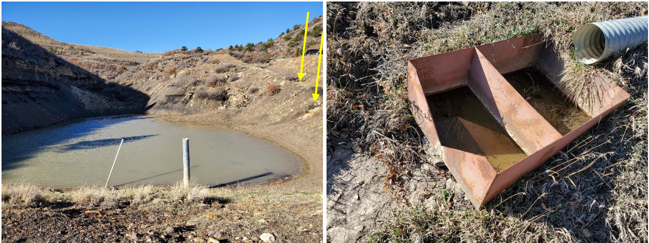
Photo 3: (Left) Pond 008. Arrows point to erosion on the pond's west bank, coming down from the path to the pond below the road. (Right) nearly full flume at Pond 008 outlet.
