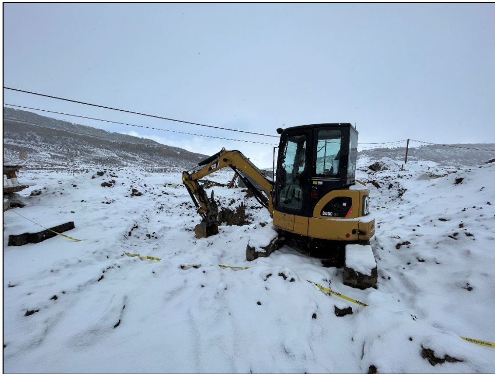
Photo 6: A water line was recently replaced behind the warehouse, the leak has been fixed, but the new line still needs to be buried.
