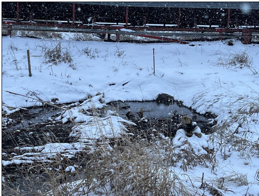
Photo 9: Discharge culvert for Pond D, cattails were recently blown down by winds.
