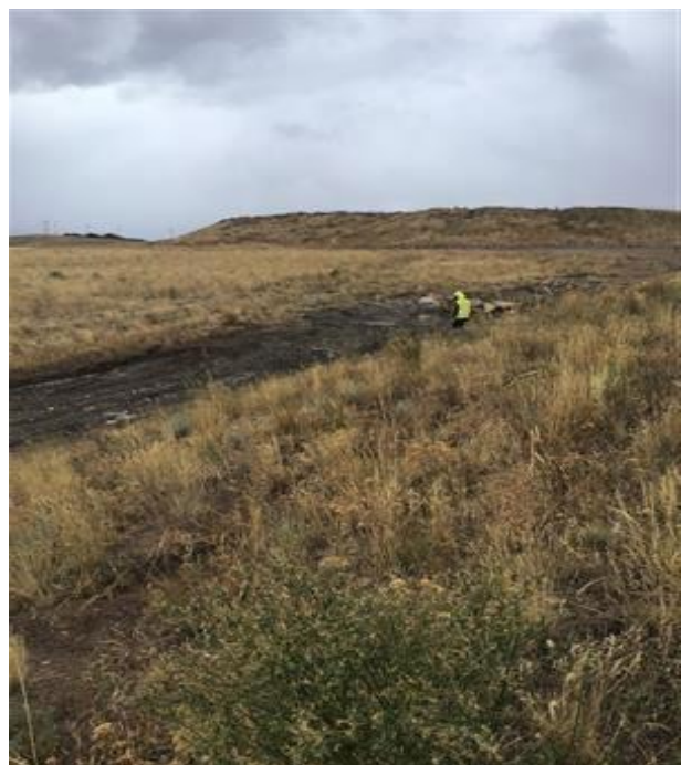
Photo 3: Recently repaired reconstructed drainage MF3 in parcel LA18, with check dam in upper right.
