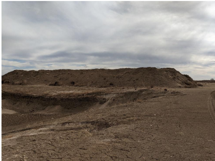
Backfill material stockpile.
