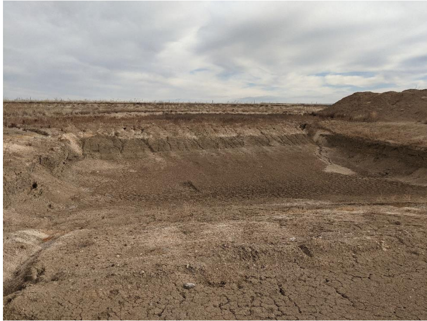
Current pit area.
