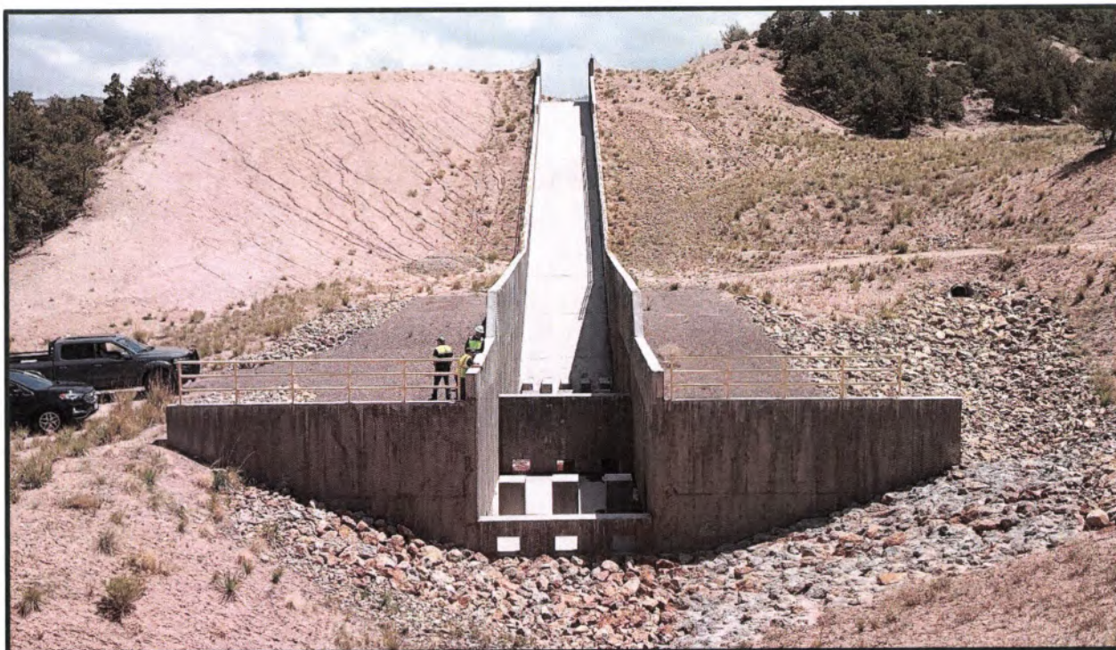
Photo 15 Looking northeast at the drop structure from the bottom, showing good conditions except for the erosional rilling along the sides.
