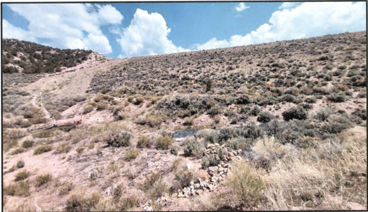
Photo 7 Looking northeast from the center at the toe, showing good conditions of the downstream face. Note the underdrain outlet and the white pumpback line at the left center.
