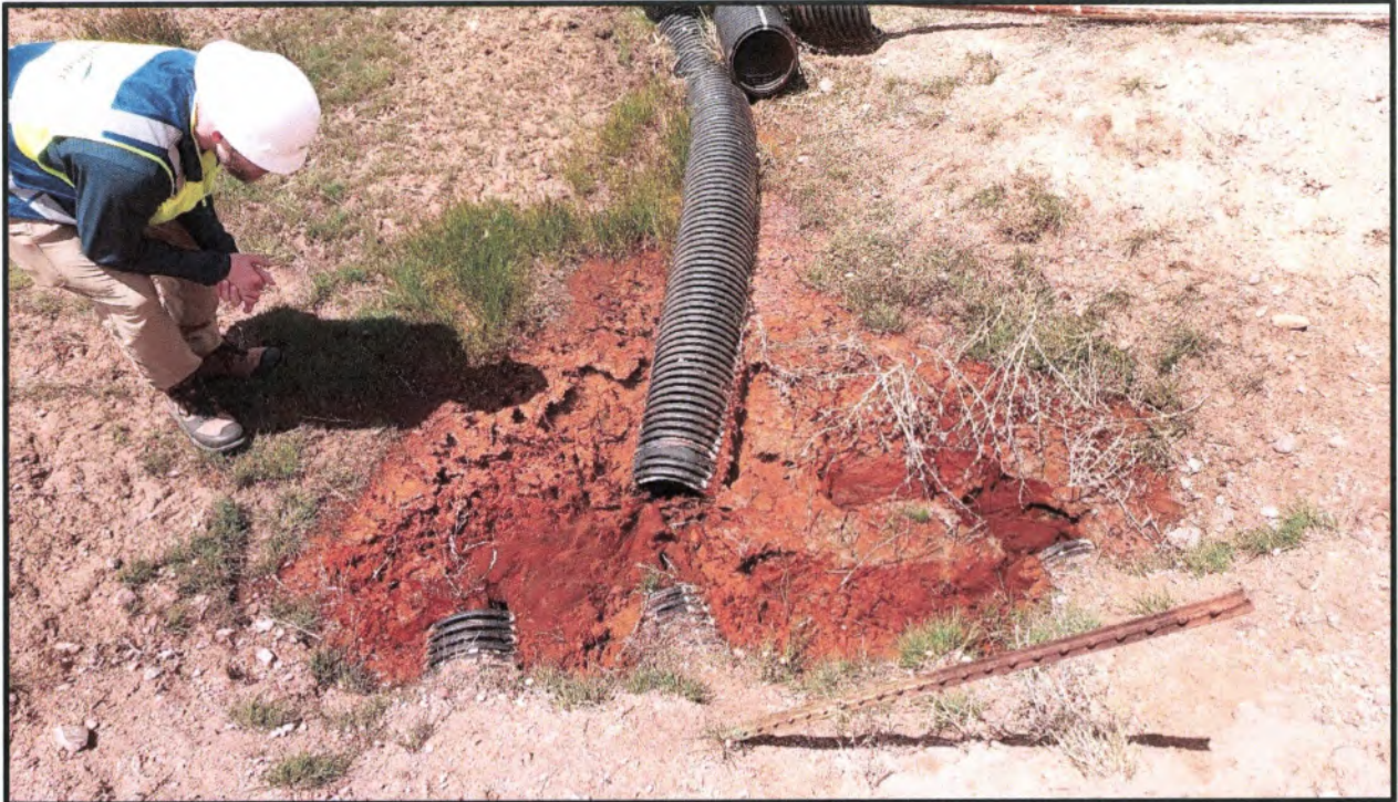
Photo 11 Closeup of the underdrain outlet pipes, showing clear seepage, low flow, and generally good conditions.
