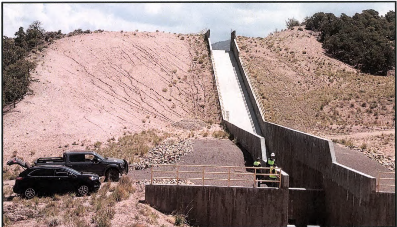
Photo 18 Looking east along the right (north) side of the drop structure, showing progression of erosional rilling and gullying on the slope face.
