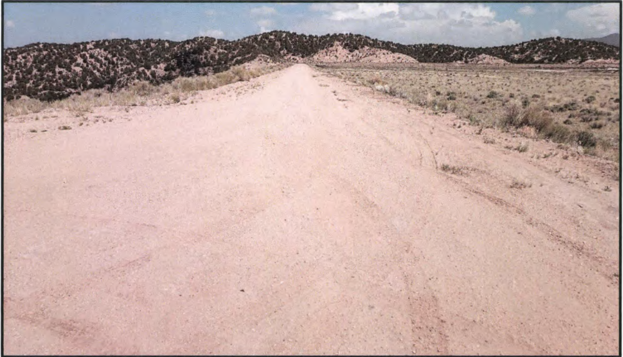
Photo 5 Looking north along the dam crest, showing good conditions and straight alignment.
