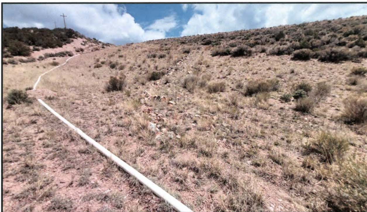
Photo 10 Looking northeast over the right downstream groin and rock drop channel, showing good conditions. Note the white pumpback line at the left.
