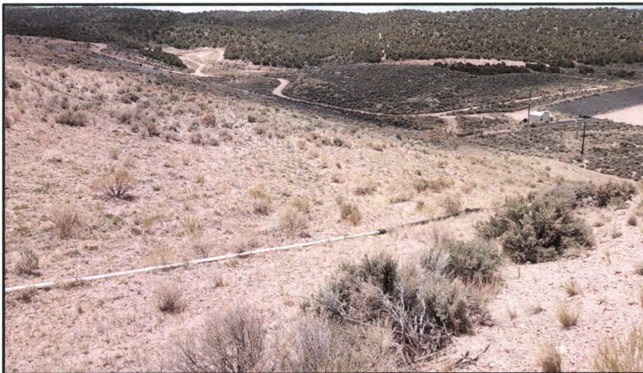
Photo 9 Looking south over the right downstream groin, showing significantly improved revegetation conditions following 2013/2014 erosion repairs. Note the seepage collection pond at the upper right.
