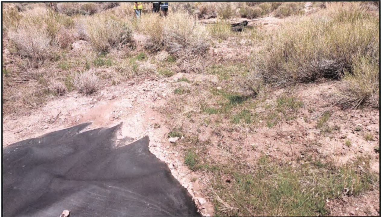
Photo 12 Looking north at the lower end of the HDPE left downstream toe runoff channel, showing near complete blockage of the culvert (upper middle of photo) with sediment.
