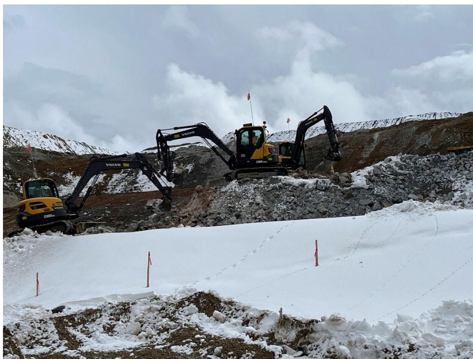
March 13, 2024 – Removal of ROM material up 2:1 slope.
