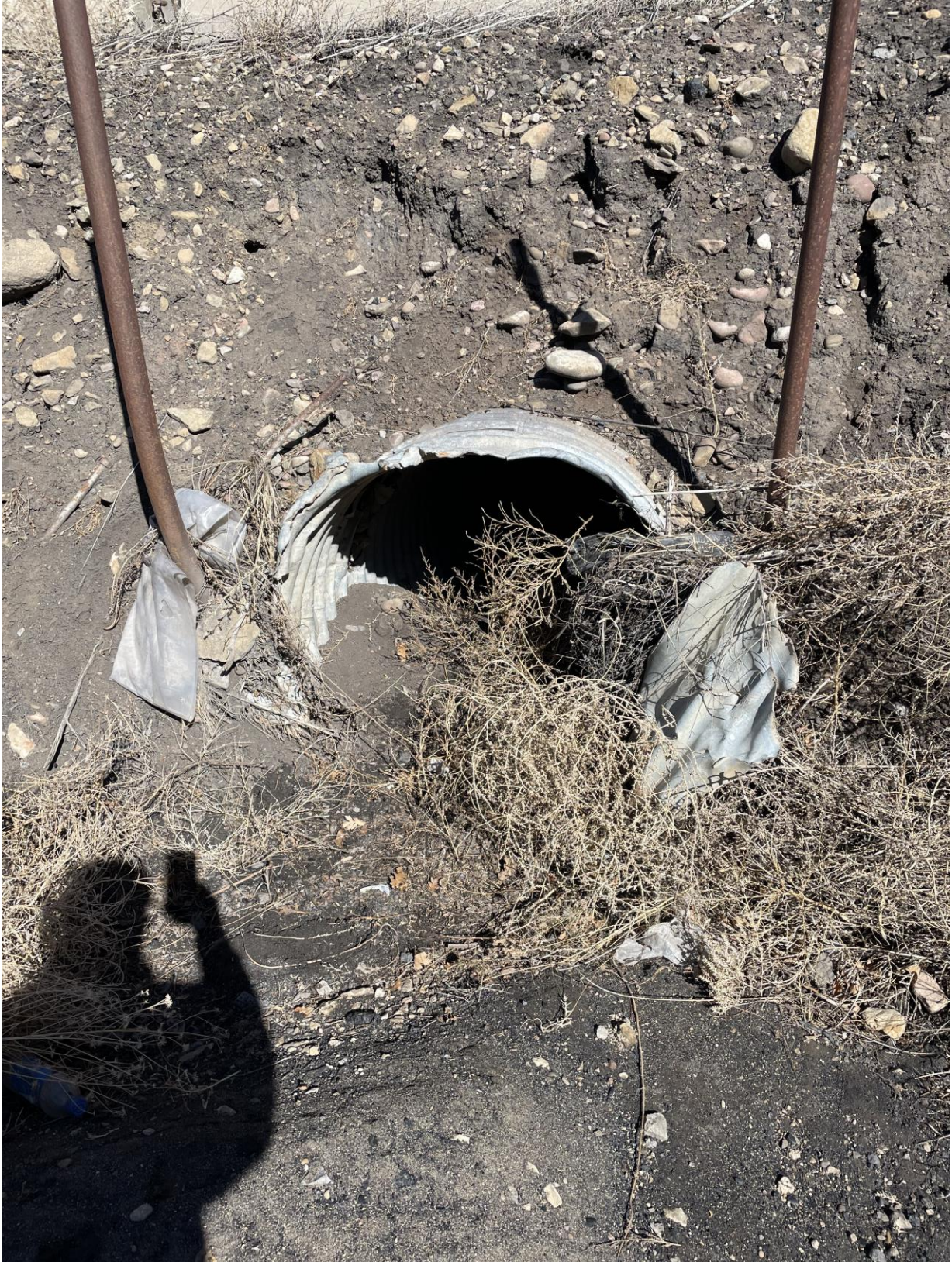
Picture 03 – C-32 with damaged inlet
