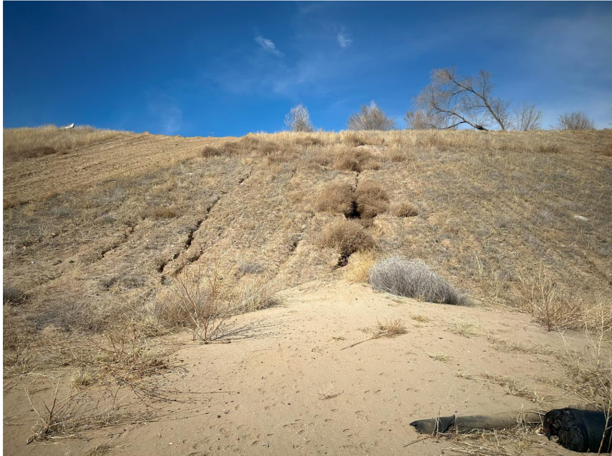
Photo 5. Erosion gullies in central area of buttress, note sand at toe of slope
