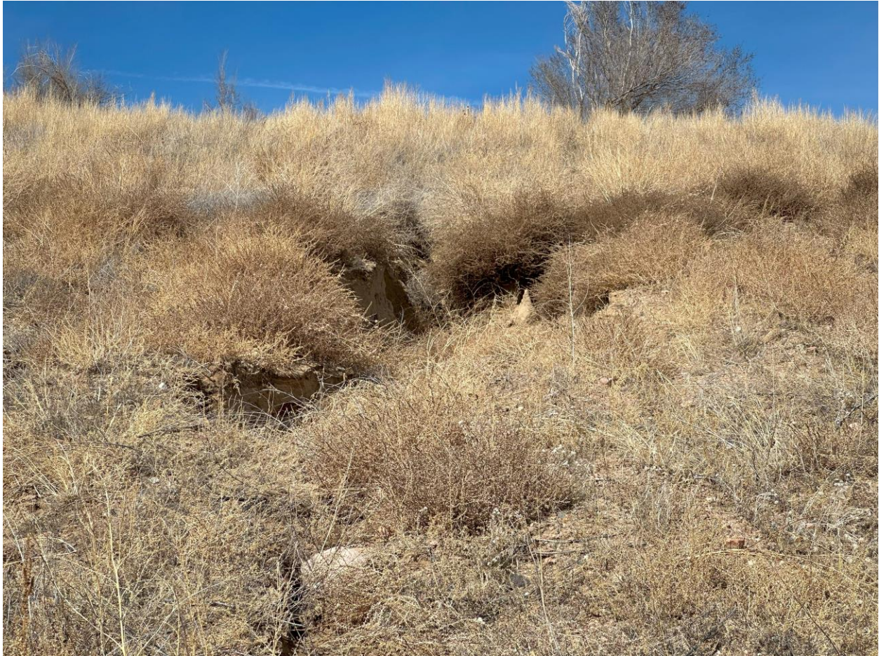
Photo 4. Erosion gully in eastern portion of buttress
