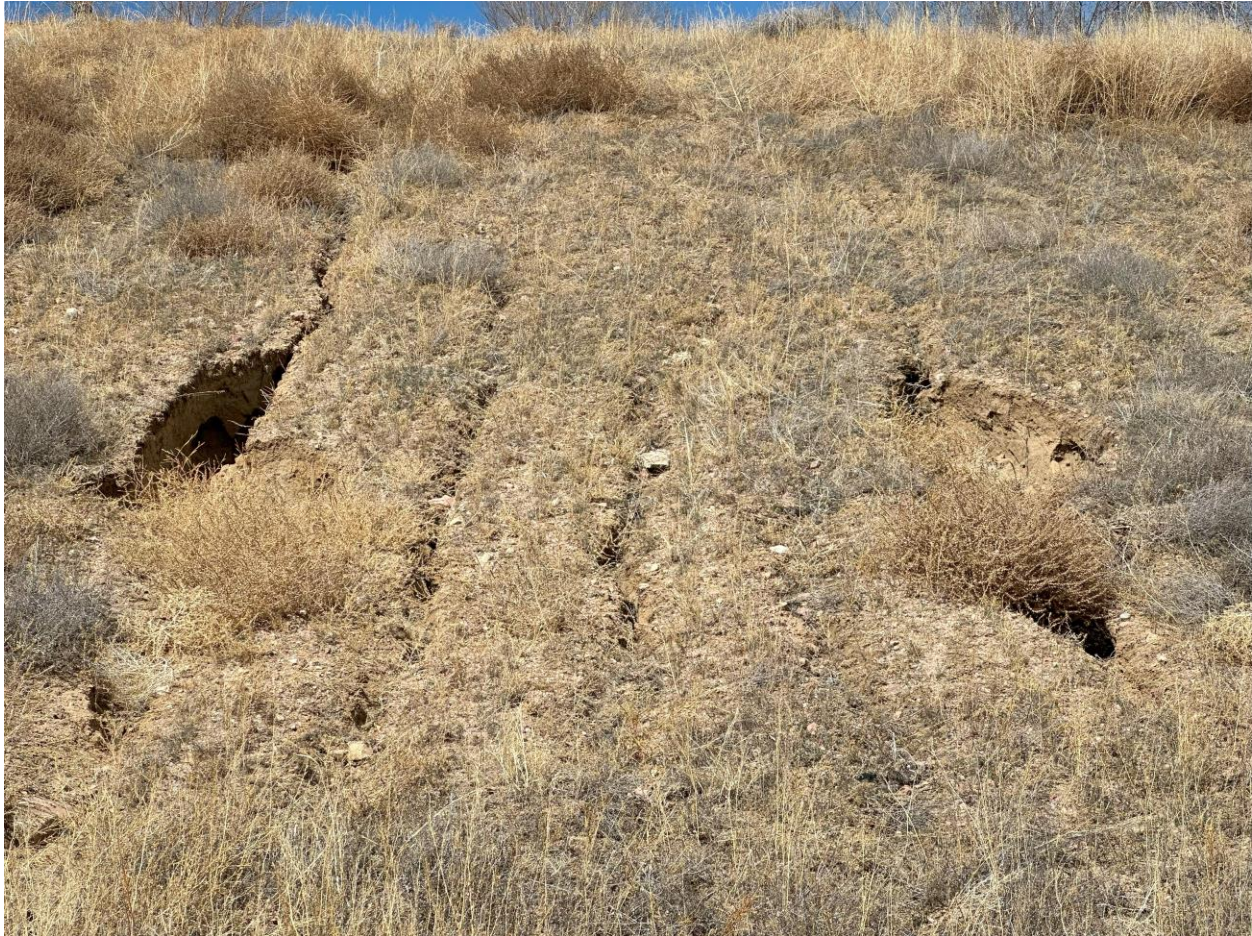
Photo 6. Erosion gullies in central area of buttress
