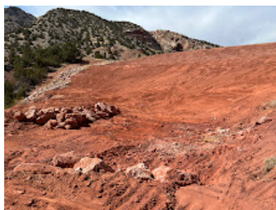
Fremont Quarry Repair 001.JPG 10288K
