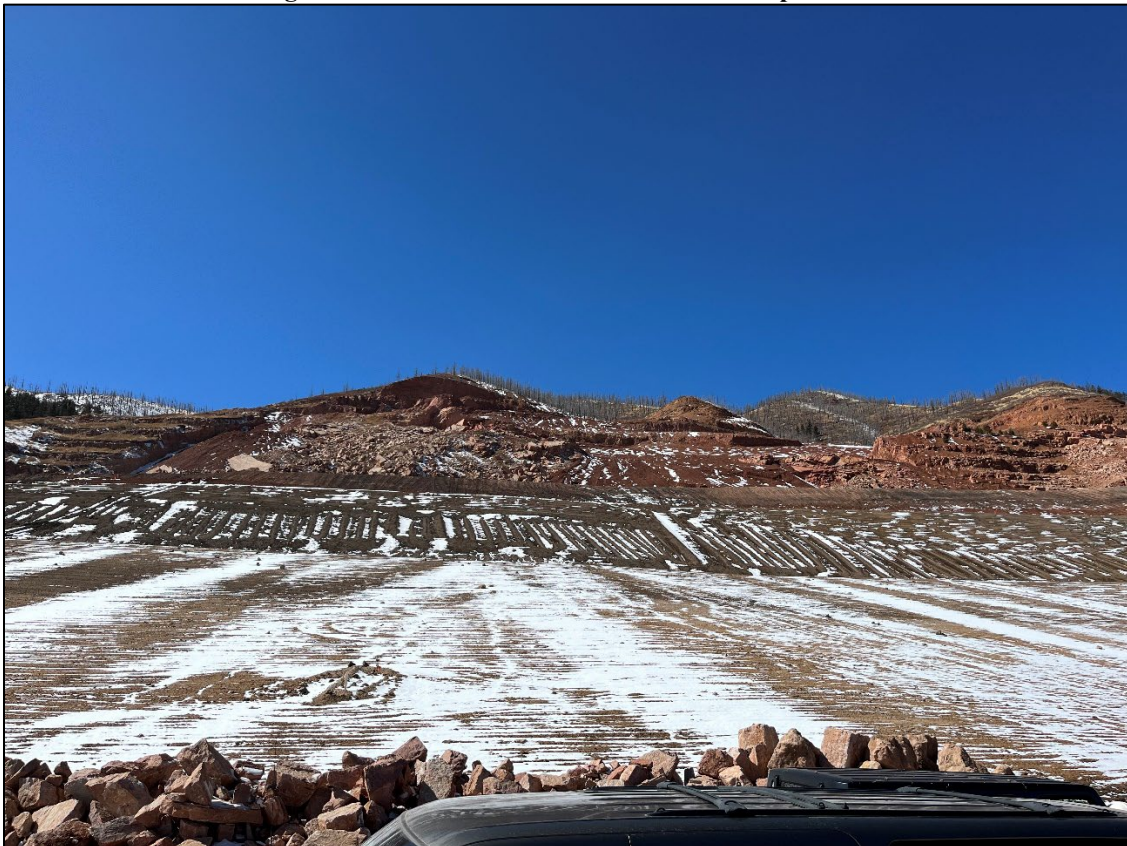
Photo 2: View west of the benches, each in various stages of backfill and topsoiling.
