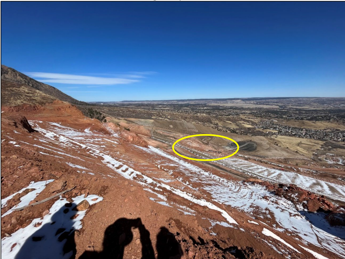
Photo 8: View northeast of the benches in progress, a channel will cut through this area to drain water from the mountain seep away from the benched area, the 'Dragons Back' is visible to the east (circled).
