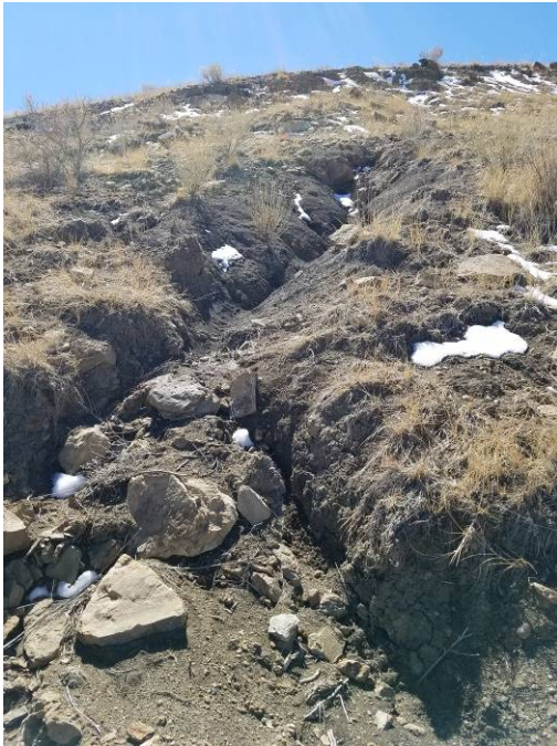
Figure 4. Rill above ditch D11.
