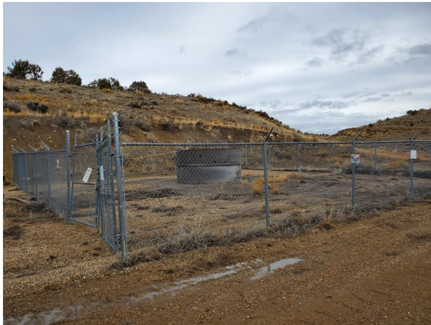
Photo 8 – B Seam Vent #1. Fence prohibits unauthorized entry and pad shows no signs of instability.
