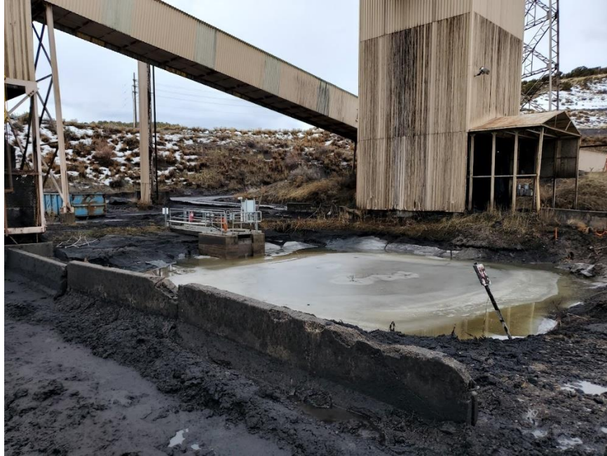
Photo 3 – Pond PP-1 near the prep plant. No signs of erosion or instability. Water level lower than previous inspection.
