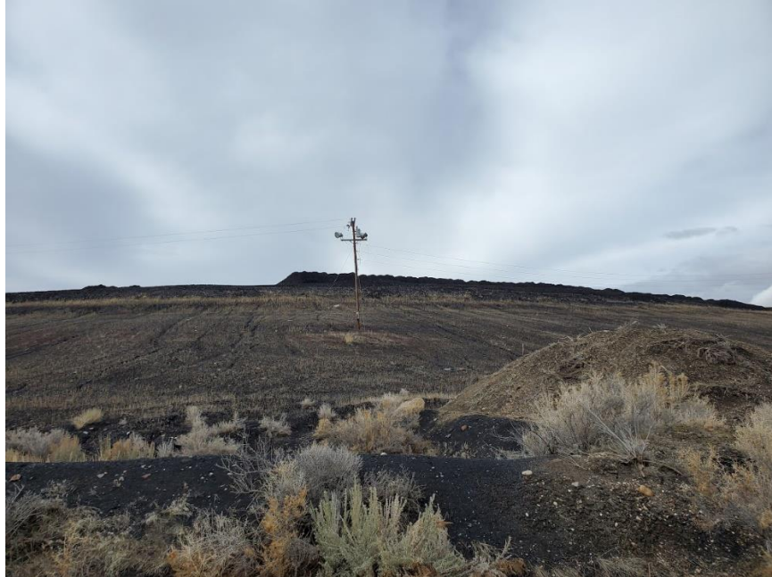
Photo 7 – Waste Pile RP-2/3/4 with minor rills on the slope face. Windrows can be seen on top of the pile.
