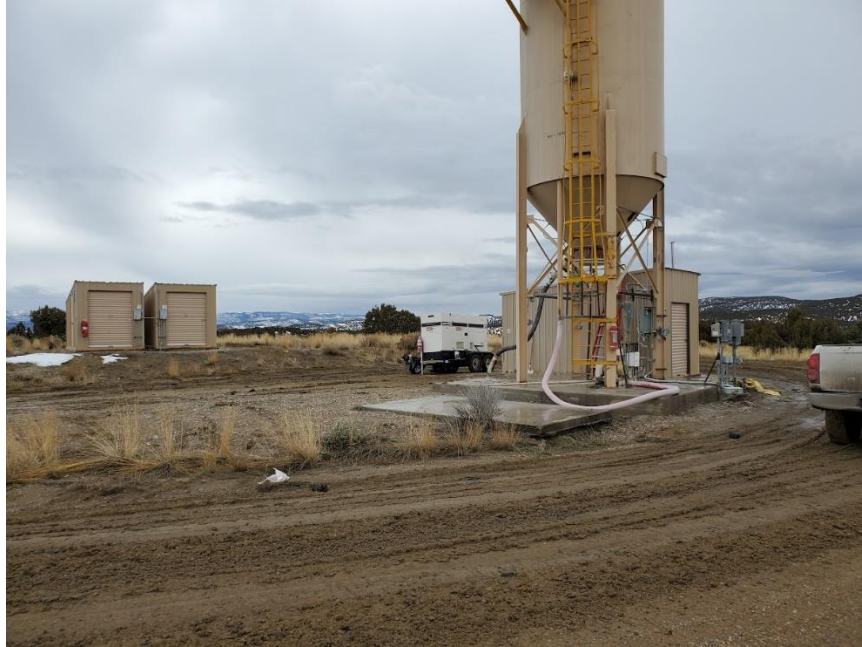
Photo 9 – RDH-2 pad and rock dust tank. Pad shows no signs of instability.
