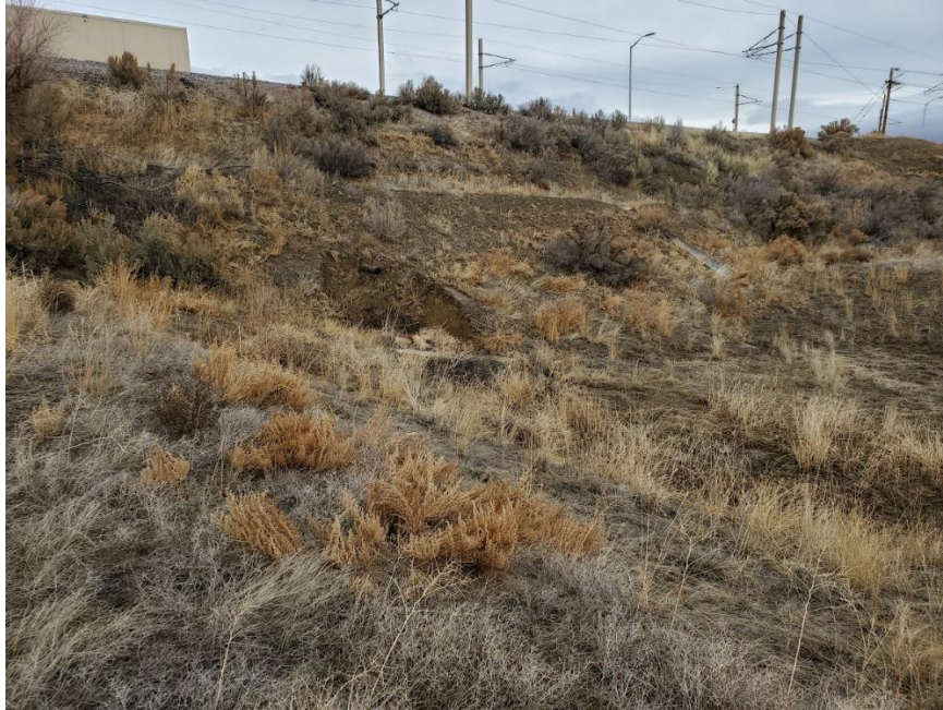
Photo 5 – Erosion scar in pond RR-1. There appears to be no change from previous inspections.
