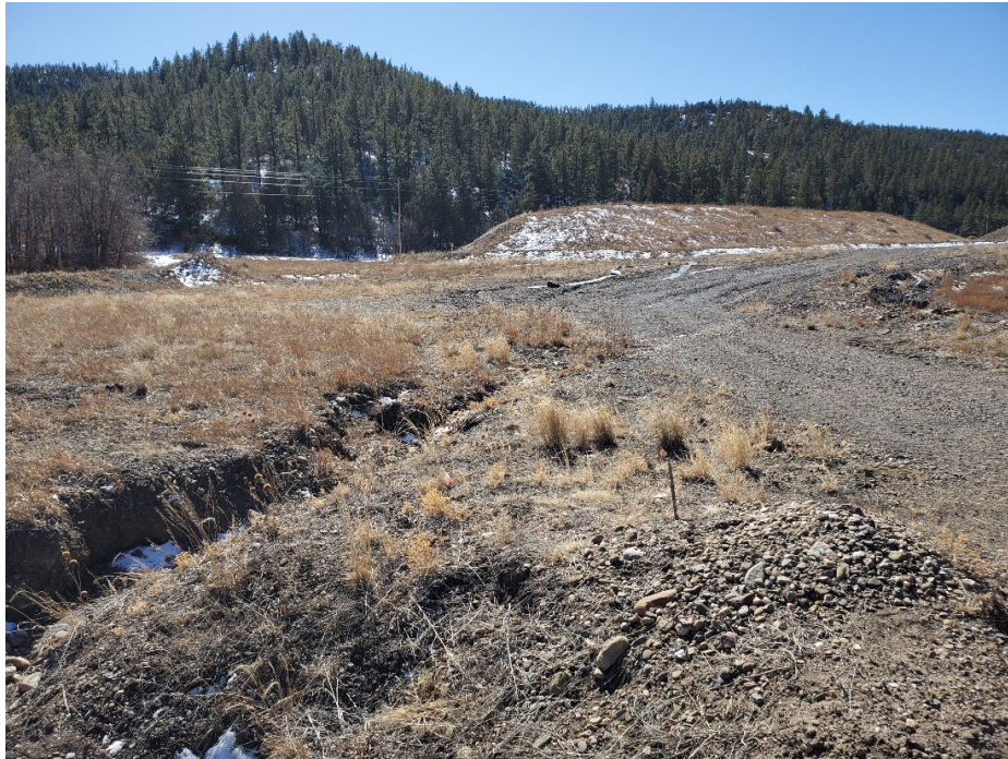
Photo 9: Erosion from surface water run-off flowing to the north-east from the flat-road-area of the Stockpile Storage Area (to the east of the Train Yard).
