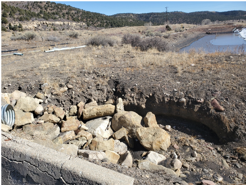
Photo 7: Scouring around outlet of C65.
