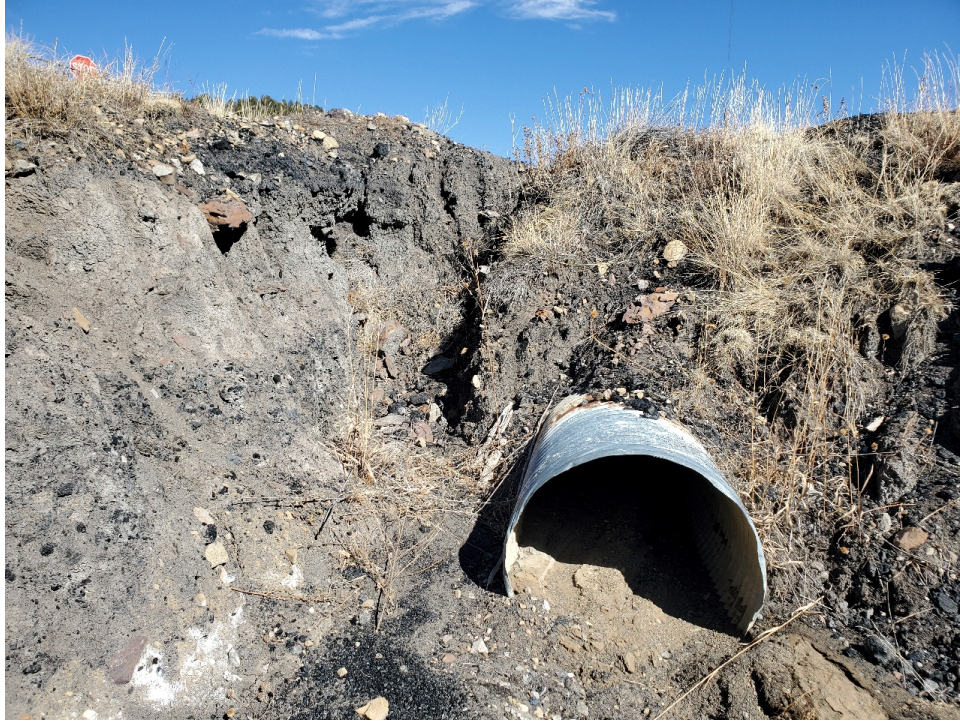
Photo 2: Erosion leading down from north side, near the highway at culvert C14. The sediment also needs to be cleaned out of C14.
