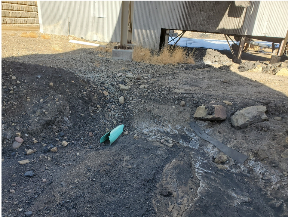
Photo 5: The broken green PVC pipe is in the location of culvert C31A on Map 13. It appears that this culvert is no longer functional or functioning as intended.
