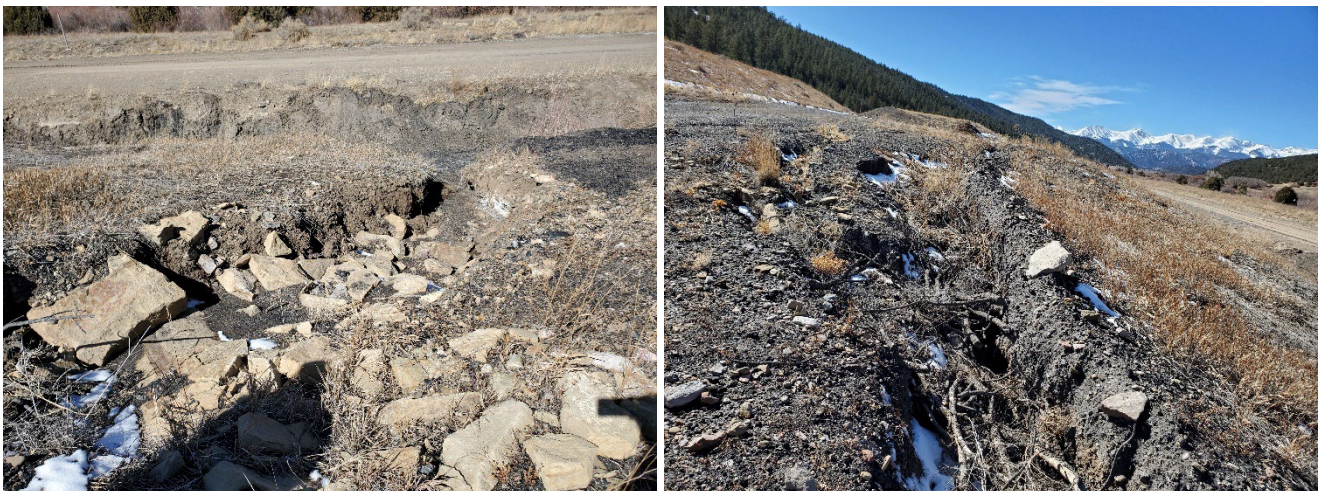
Photo 10 (A and B): Erosion from surface water run-off flowing to the north from the flat-road-area of the Stockpile Storage Area (to the east of the Train Yard). The Operator stated that they had tried to armor the gully with check dams (A) and branches (B) but they have since failed.
