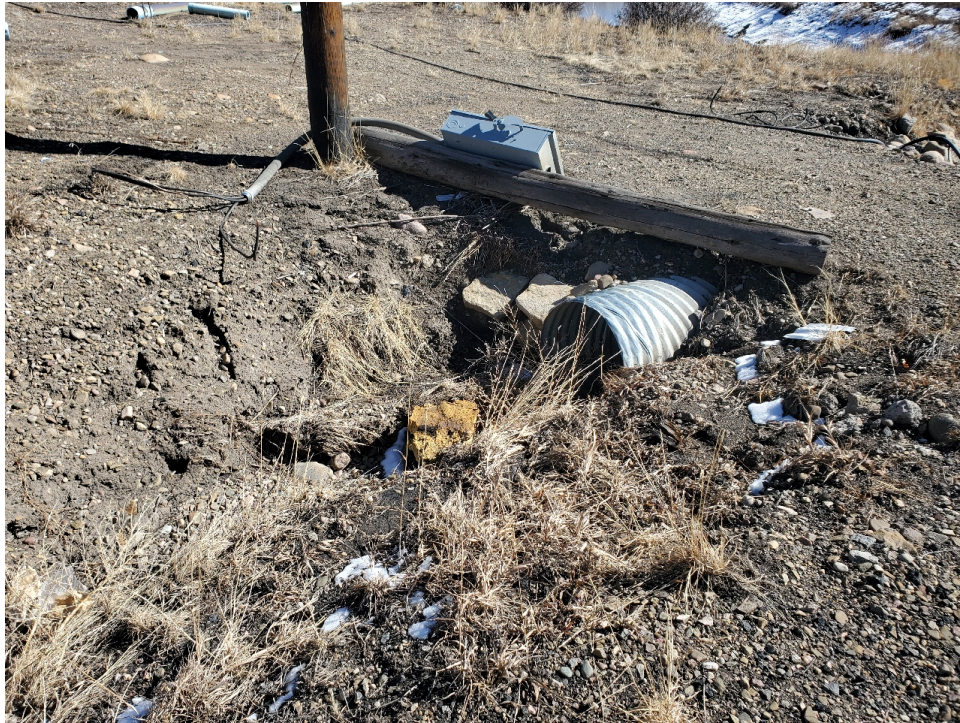
Photo 6: Scouring around inlet of C65
