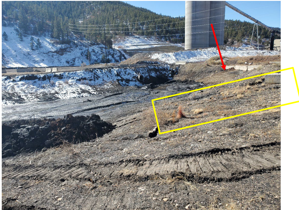
Photo 8: Arrow indicates where erosion leading under the concrete berms next to the road has been repaired and Pond 007A's western bank. The portion of the bank (within the rectangle) still requires some repairs.
