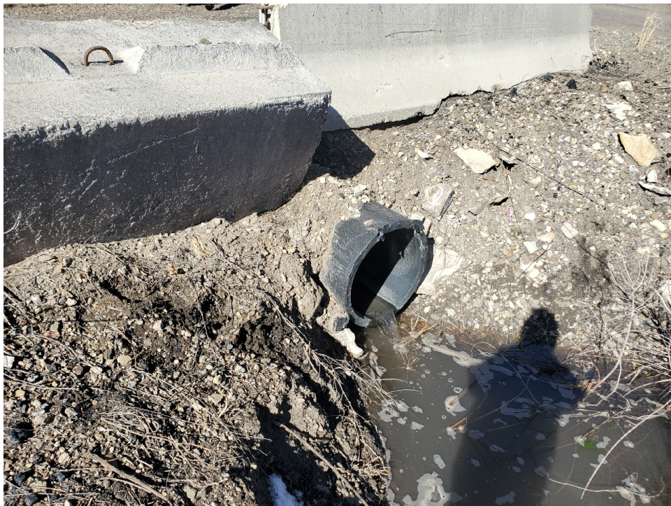
Photo 3: Erosion cutting down the side of culvert C16D.
