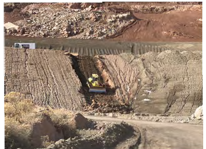
1. DOZER REPAIRING EROSION GULLY.
