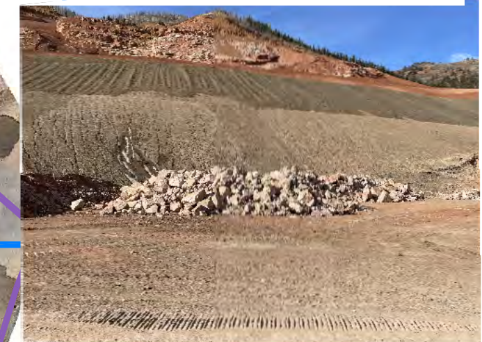
2. SCREENED GRAVEL AND RIPRAP STOCKPILE.
