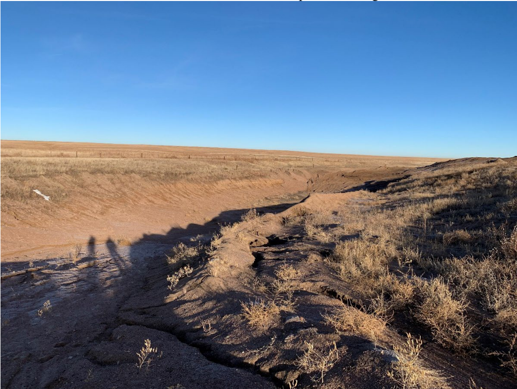
Photo 2 – Low spot in drainage that needs to be filled in.
