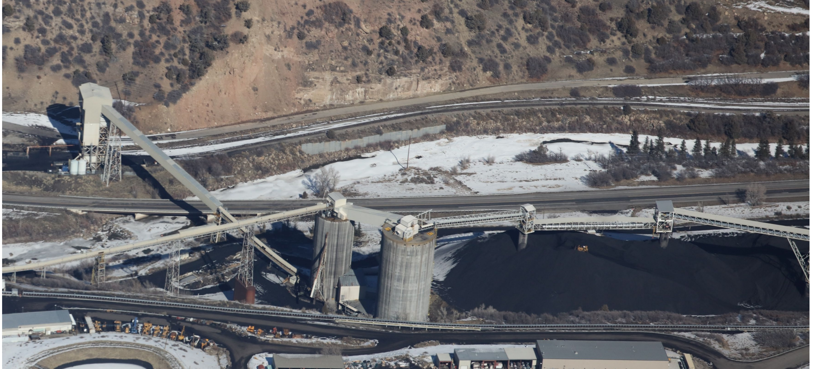
Figure 3: Clean coal stockpile, coal silos, train loadout.
