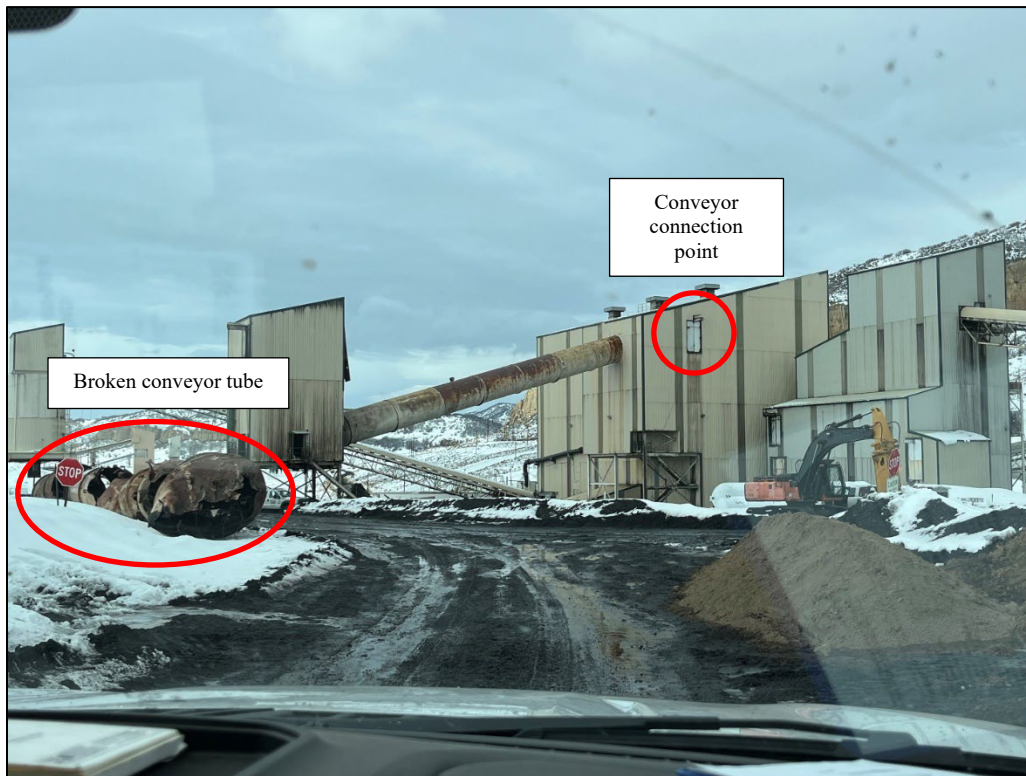
Figure 2: A conveyor tube connected to the east side of the Wash Plant was recently damaged, a temporary conveyor will be built in its place until a new tube can be fabricated.
