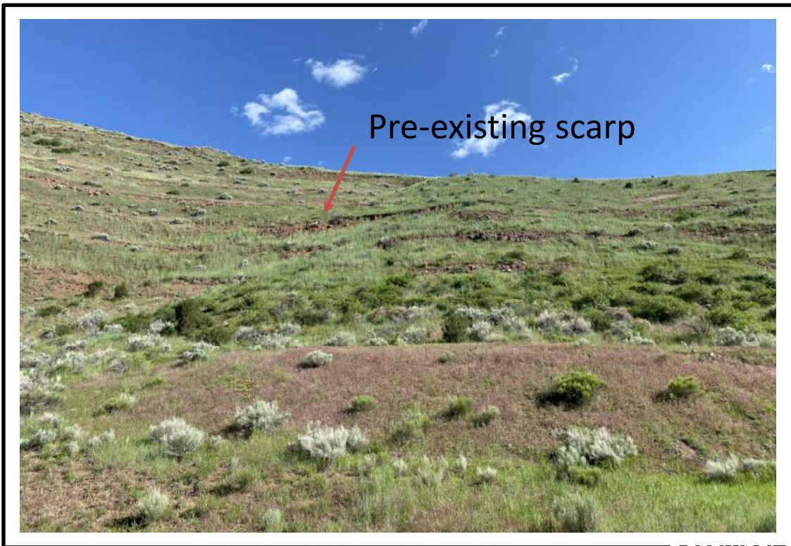
Photo 15: Looking North from Main Pit access road at pre-existing scarp on Northeast Wall 1 (June 2023)
