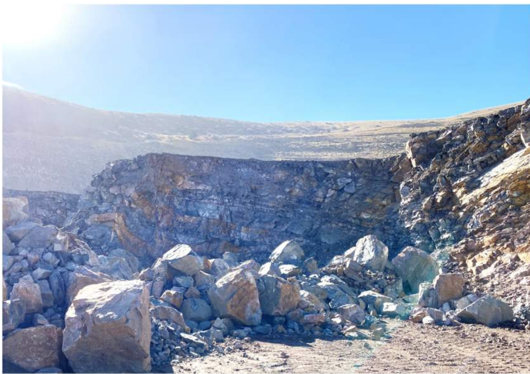
Photo 8: Looking south at fault in corner of south and west temporary excavation, Bench EL 6405 (November 2023)
