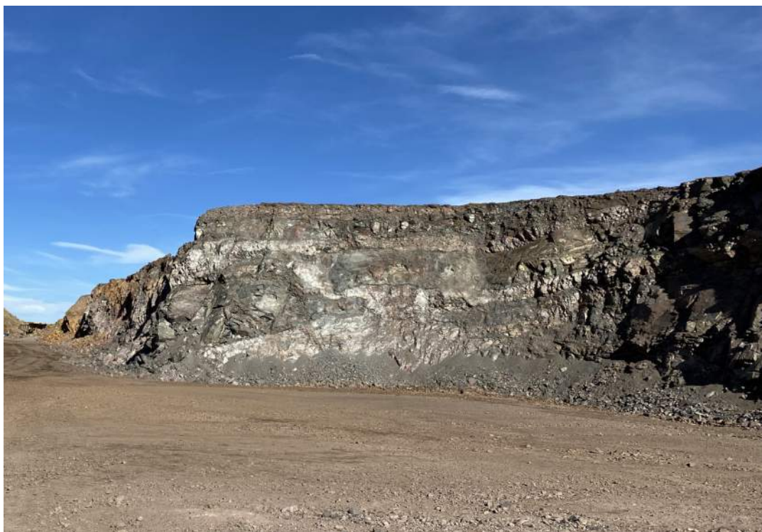
Photo 10: Looking NW at localized shear zone in east temporary excavation, Bench EL 6405 (November 2023)
