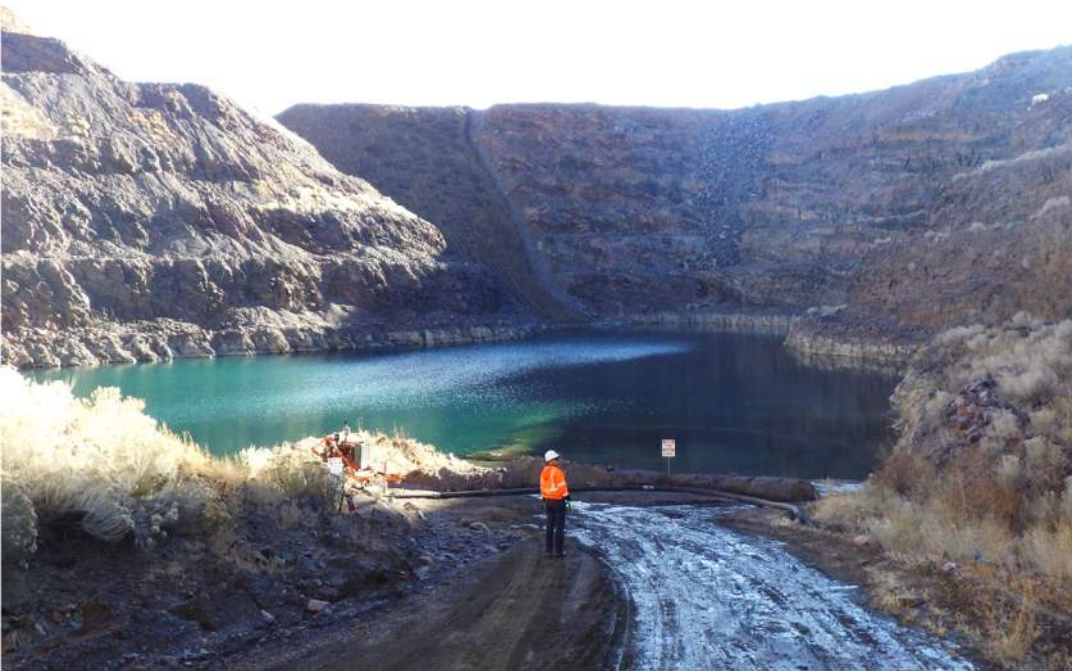
Photo 12: Looking East at Northeast Walls 1-2 (November 2023)
