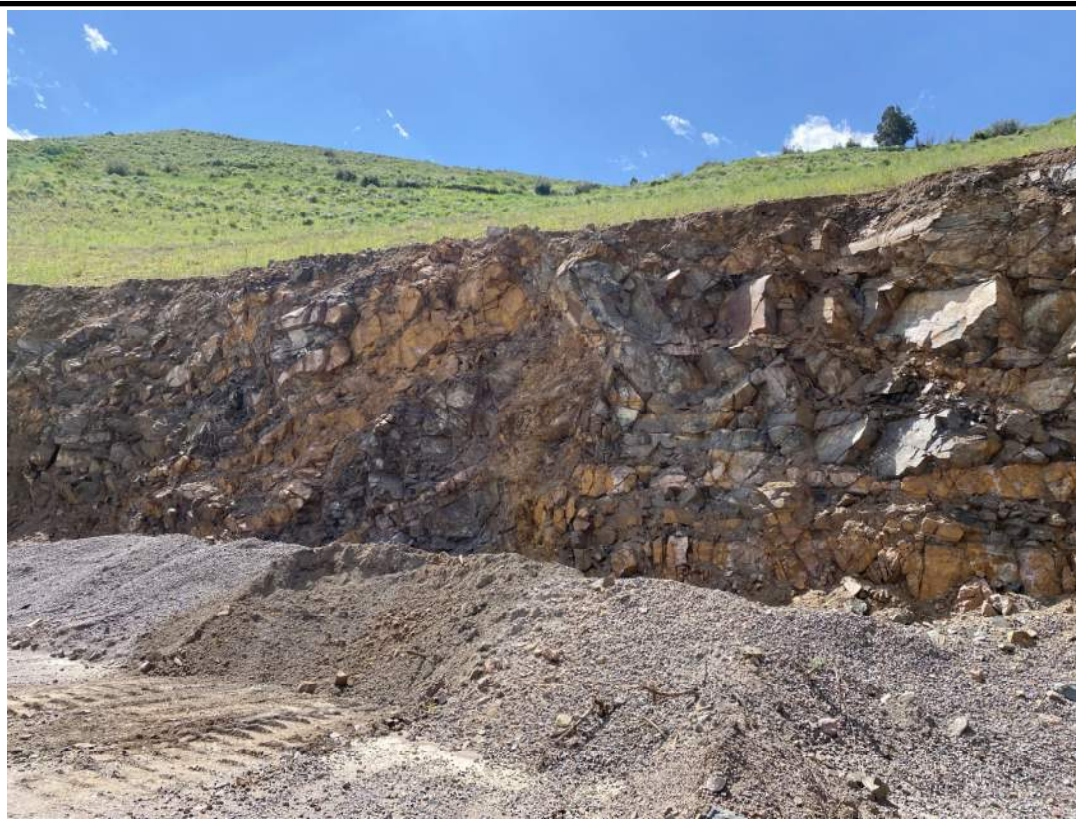
Photo 5: Looking SE at fault in Southern Walls, Bench EL 6440 (June 2023)
