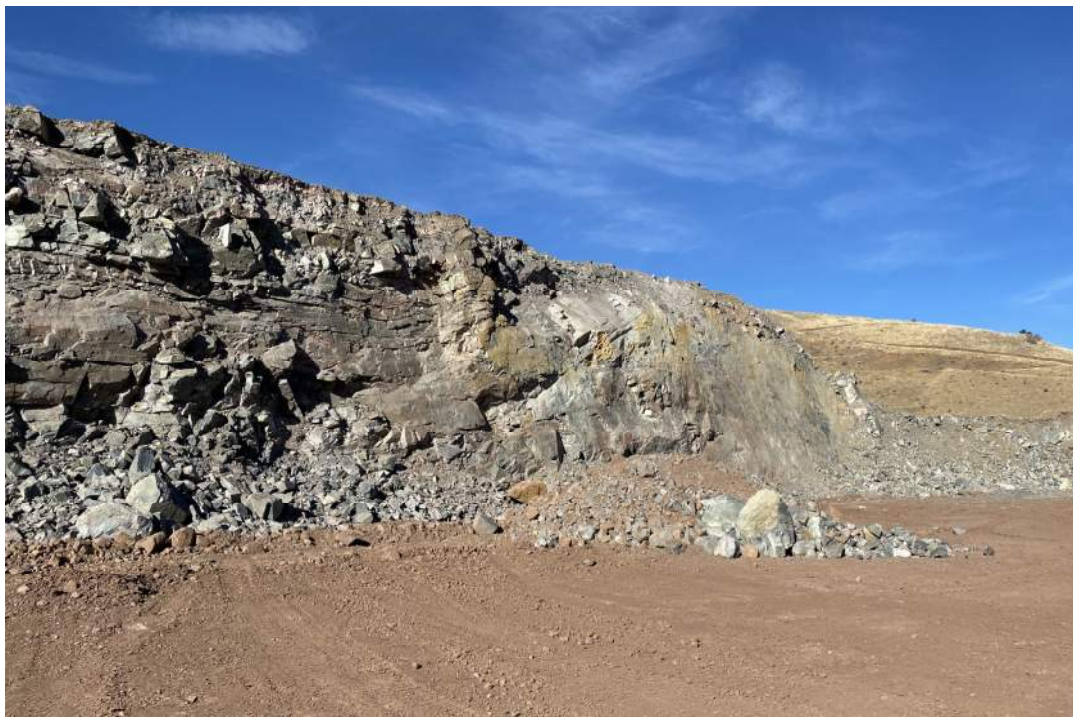
Photo 9: Looking NW at massive face of west temporary excavation, Bench EL 6405 (November 2023)
