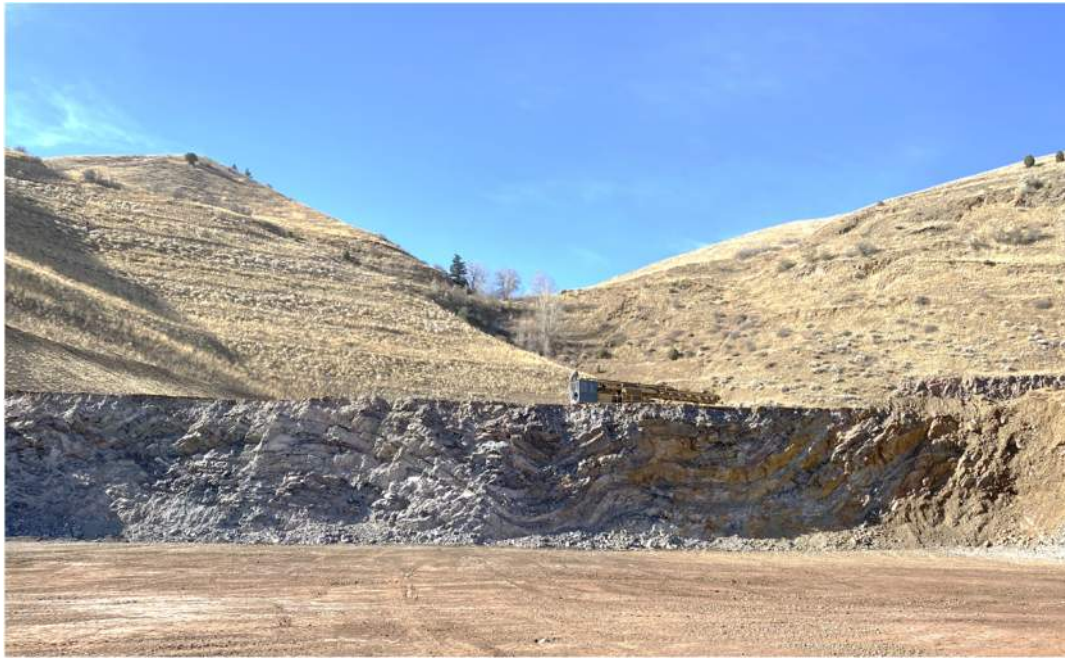
Photo 7: Looking West at folding in temporary west excavation wall, Bench EL 6440 (Nov. 2023)
