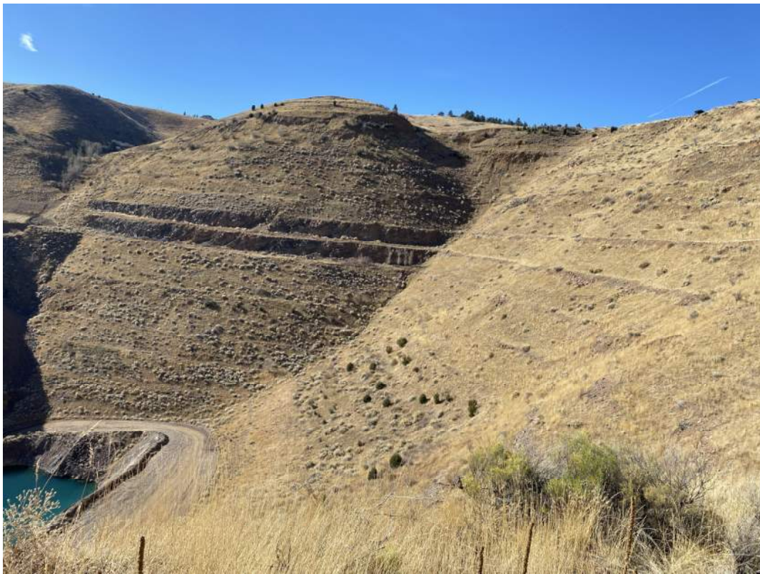
Photo 18: Looking West at Northeast Walls from top of Main Pit
