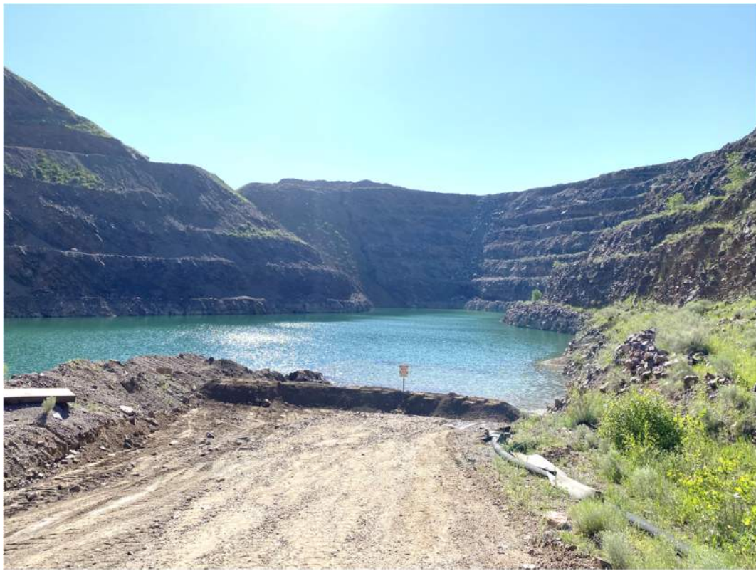
Photo 11: Looking East at Northeast Walls 1-2 (June 2023)
