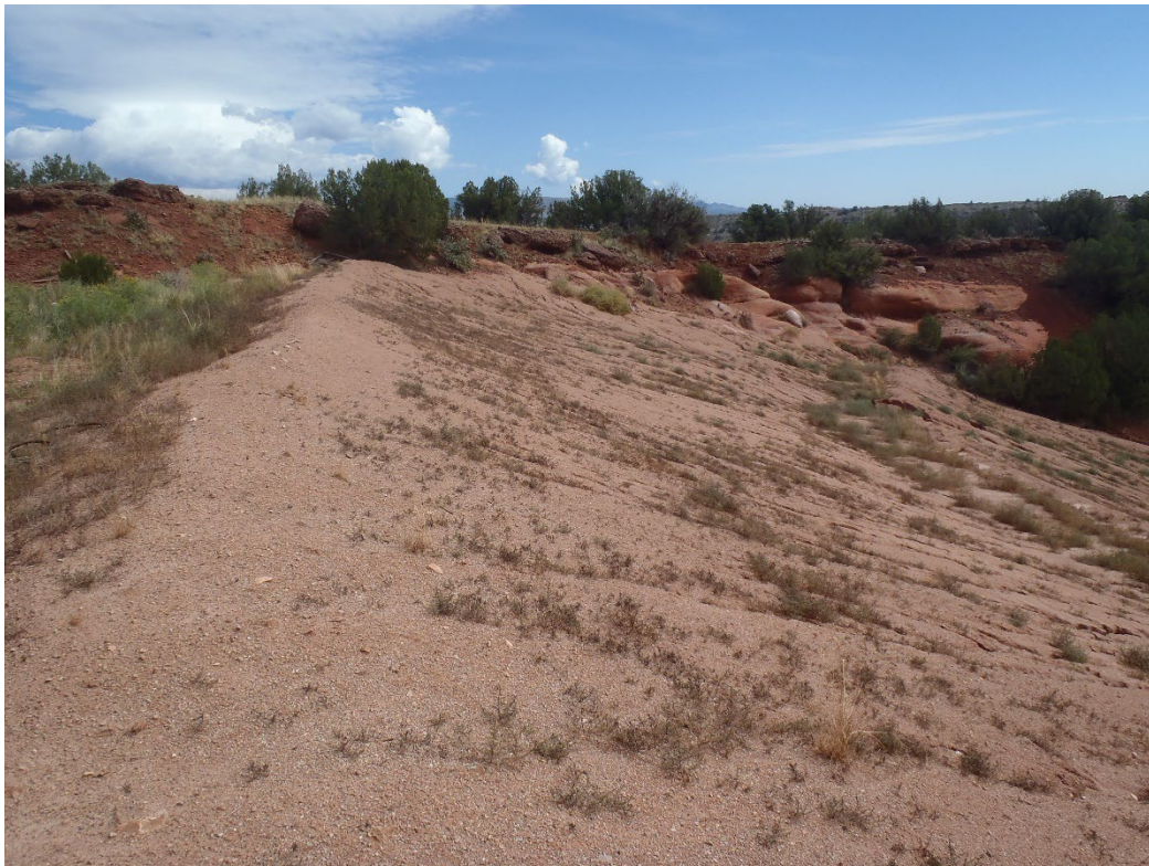
Photo 7. Upper portion of repaired Fines Disposal area (looking NE from crest).
