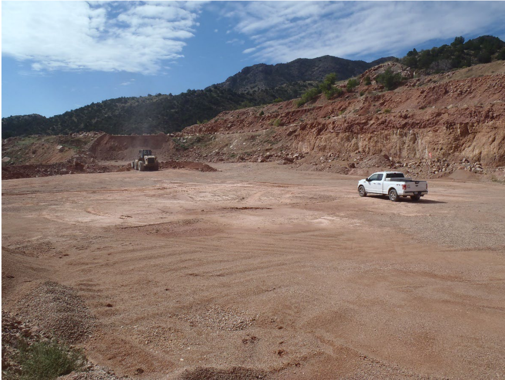
Photo 4. Pit floor (looking SSW from the east side).
