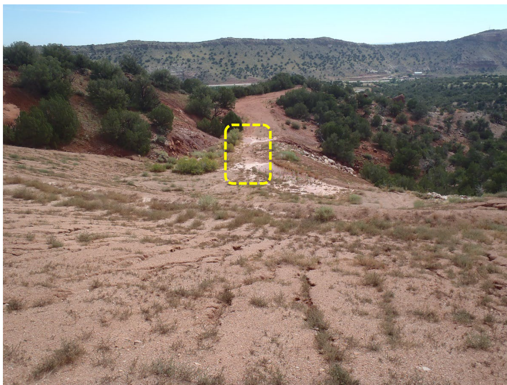
Photo 9. Lower repaired Fines Disposal area (looking east from crest) needing a sediment trap as noted.
