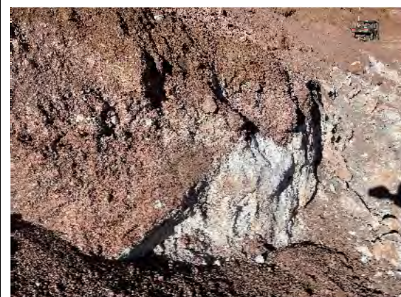
6. Mapping the fault location.
