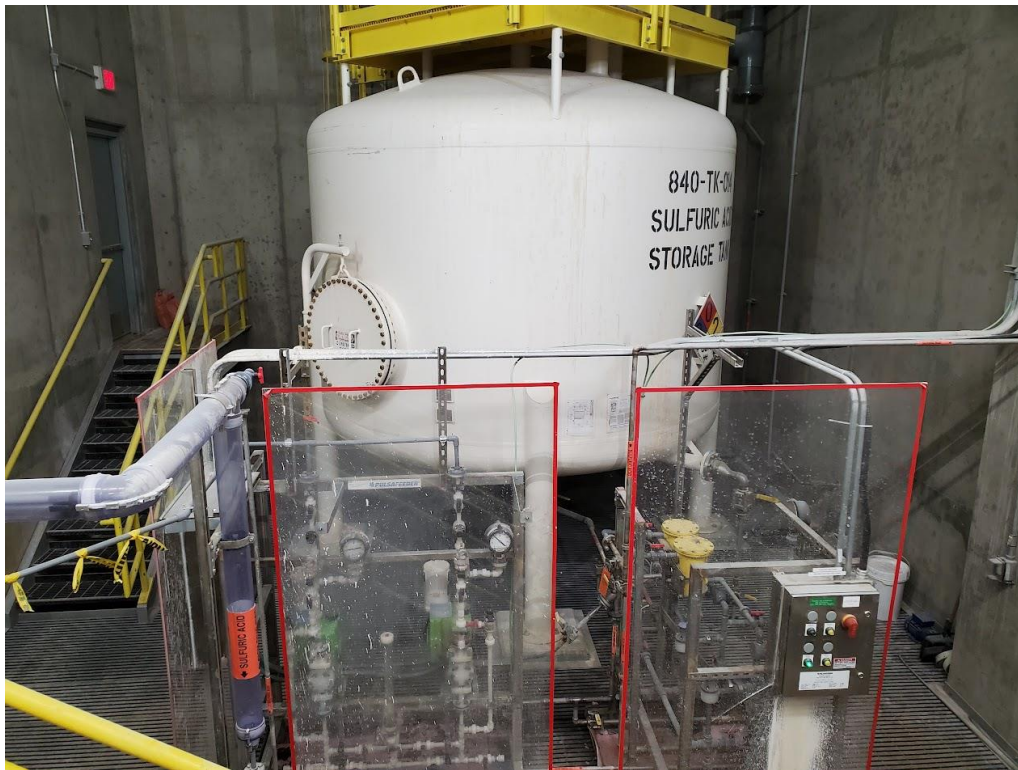
Photo 9 – View to the west of sulfuric acid storage in Filter Building of PDWTP.
