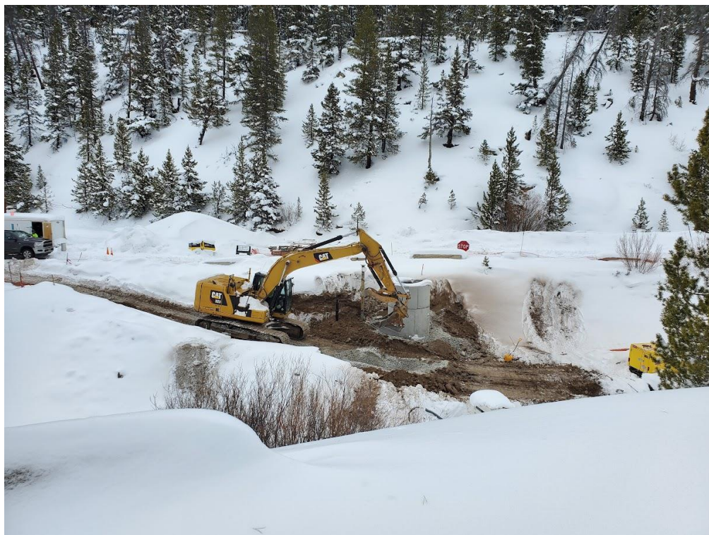
Photo 6 – View to the east of progress at 5 Dam Seepwater Collection System. Excavator is packing material around the well.
