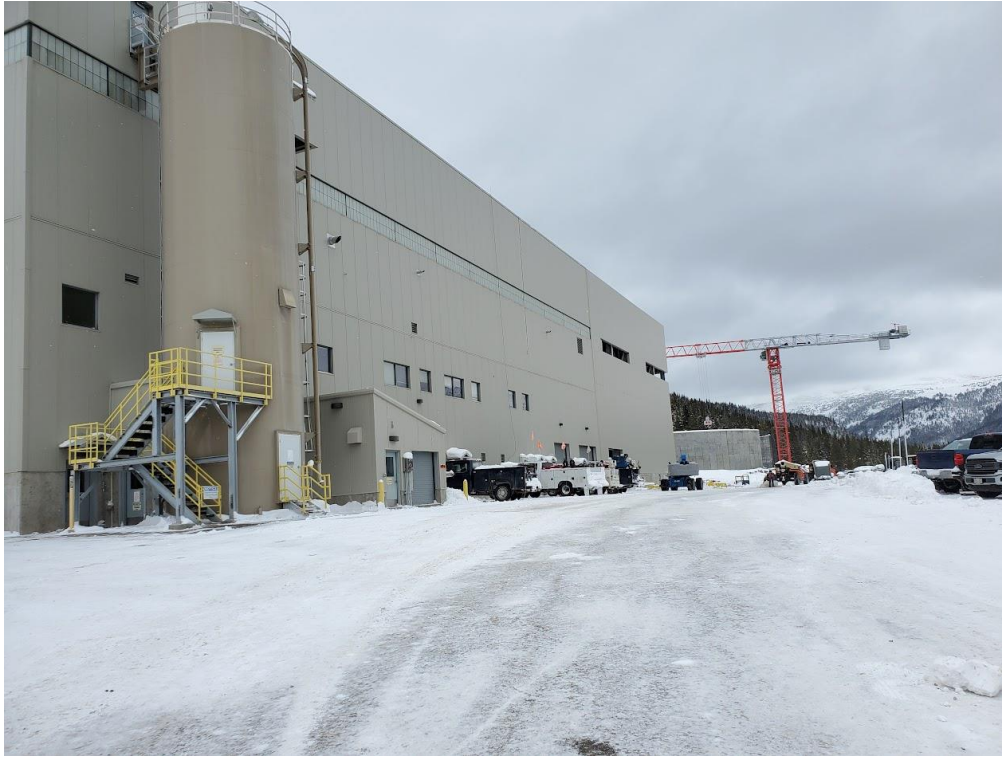
Photo 7 – View to the north of PDWTP. Lime storage can be seen in the foreground. Siding can be seen on the MRWTP in the background along with a crane that is constructing the thickener.
