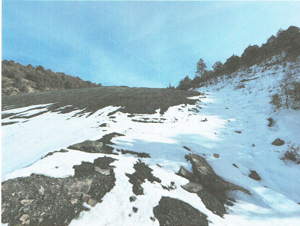
Pic. 3 – Reach 10 appears extended to top of existing pile and embankment face recompacted.
