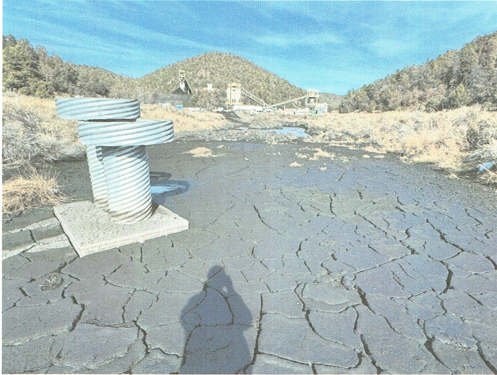
Pic. 3 Outlet structure culverts in good condition, sediment drying out.
