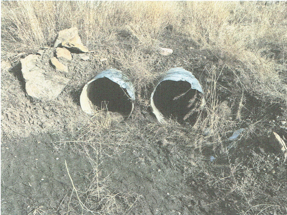
Pic. 4 –Sediment pond outlet pipes.
