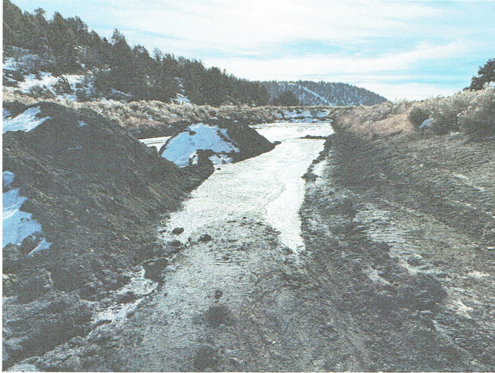
Pic. 1 – Detention Pond-sediment removal progress to date.
