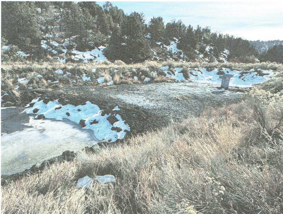
Pic. 2 – Sediment removal upstream of outlet structure allowing drying of sediment at pond outlet.
