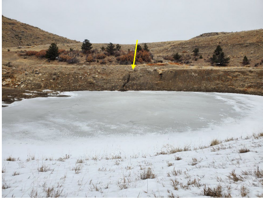
Photo 1: Rills forming on the north bank of Pond 006A.
