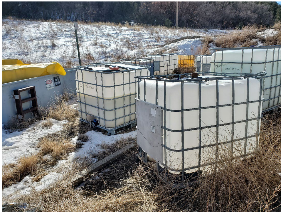
Photo 4: Portable Explosives and Chemical Storage area. The tank on the left is the leaking tank, the tank on the right is the new empty tank.
