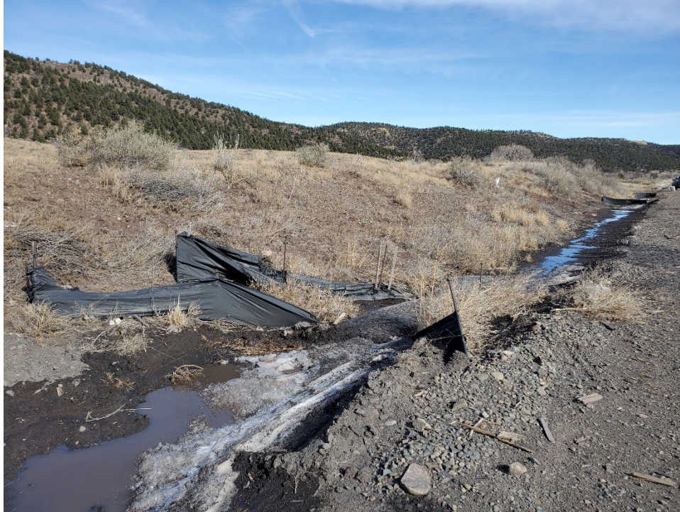
Photo 3: Western-most silt fences along the north side of the road in the SAE near Pond 007.
