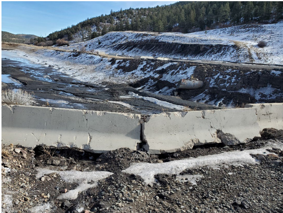
Photo 2: Erosion undercutting concrete berms along the west embankment of Pond 007.
