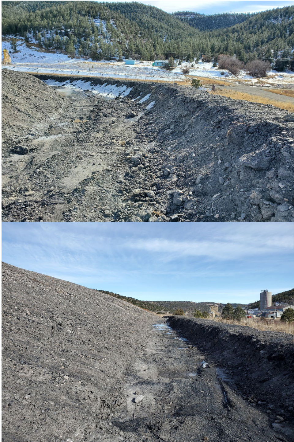
Photos 1A and 1B: 1A) Berm along the west side of DWDA#2. 1B) Berm along the south side of DWDA#2. Rills smoothed out along the bottom portion of the slope on the DWDA#2.
