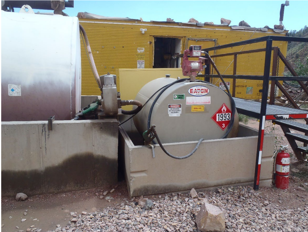
Photo 1. Diesel fuel tanks with secondary containment (processing area).
