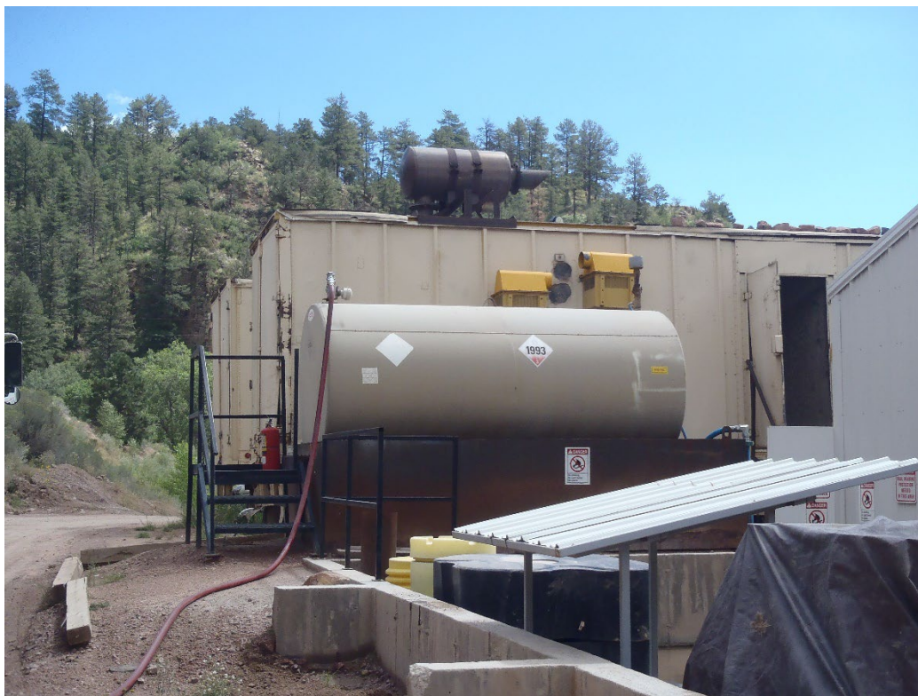
Photo 2. More petroleum tanks with secondary containment (processing area, note drums and spill kits in the foreground).
