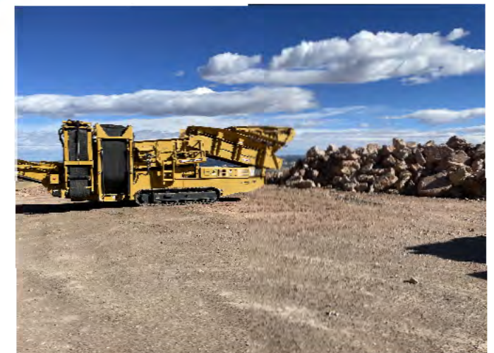
1. Astec sorting riprap.
