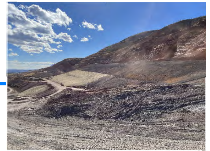
3. First bench seen from North Borrow Area.
