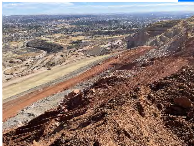
7. Compacted pit floor seen from haul road .
