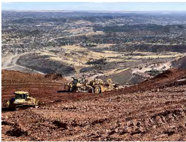
6. Dozers grading down from haul road.
