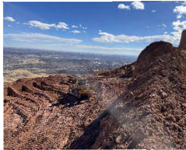
5. Dozers working near top of haul road.
