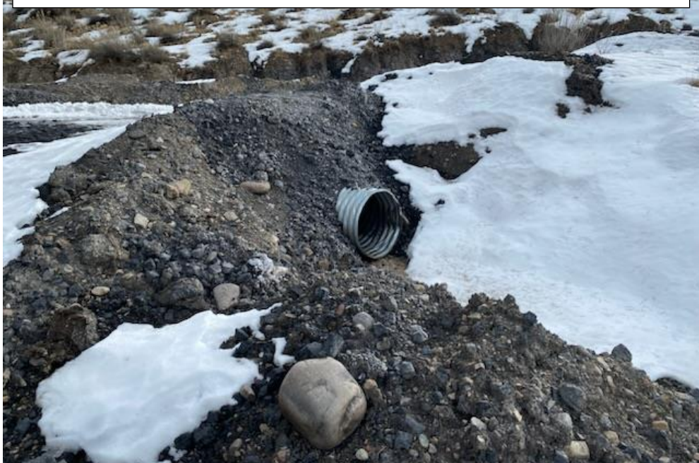
Photo 4: The lower culvert outlet along the Haul Road In-between the URDA and LRDA.
