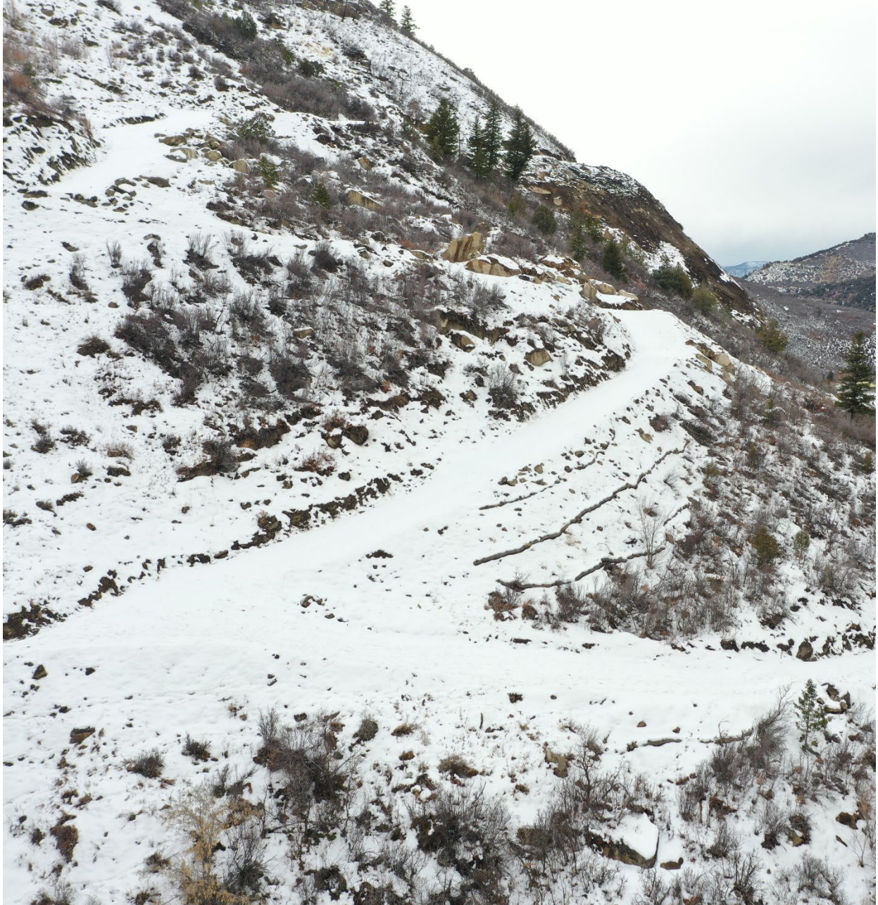
Figure 4: Upper road, with sediment control on downslope side
