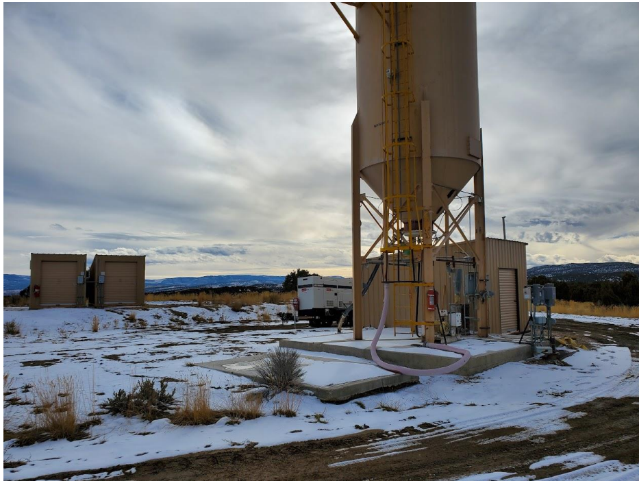
Photo 10 – RDH-2 pad and rock dust tank. Pad shows no signs of instability.
