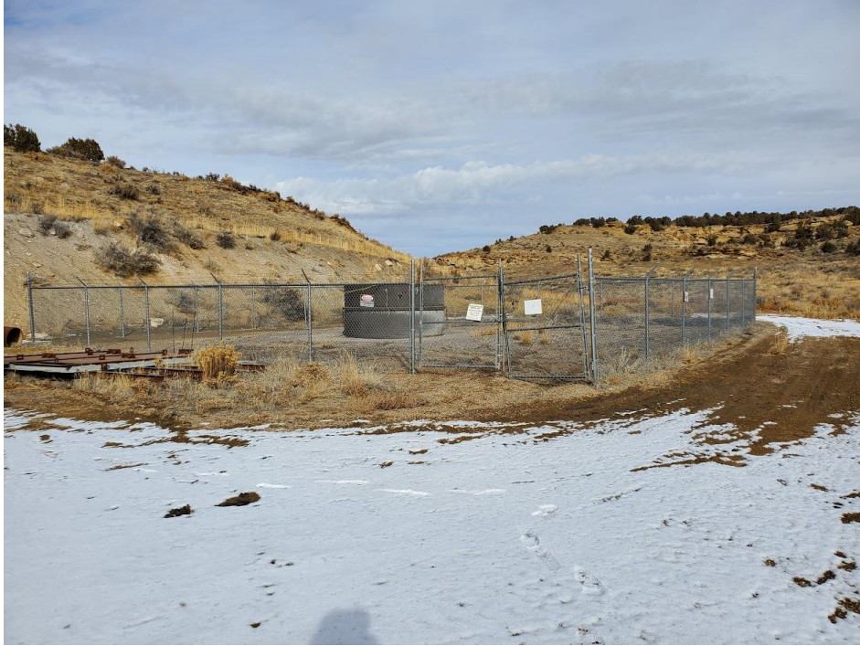
Photo 9 – B Seam Vent #1. Fence prohibits unauthorized entry and pad shows no signs of instability
