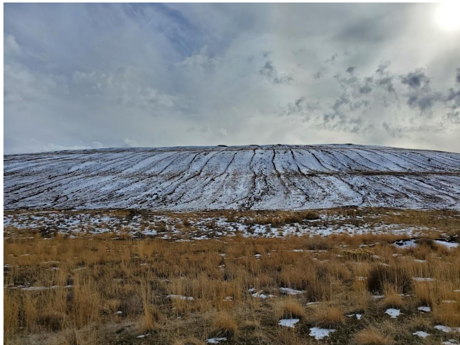
Photo 56– Waste Pile RP-2/3/4 with minor rills on the slope face.
