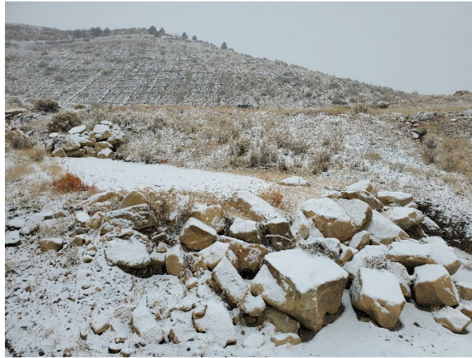
Photo 4: Check dam nearly full of sediment.
