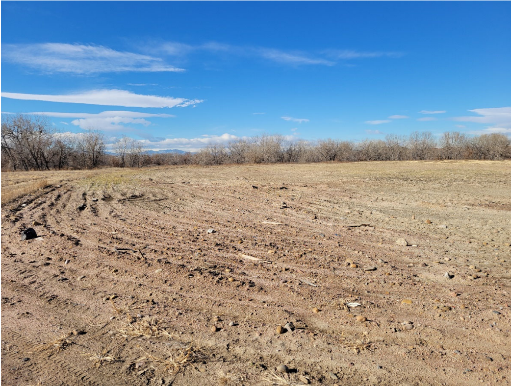
Photo 5: View looking west across recently graded area in the southwest section of the permit area. Straw mulch is thin or missing here.
