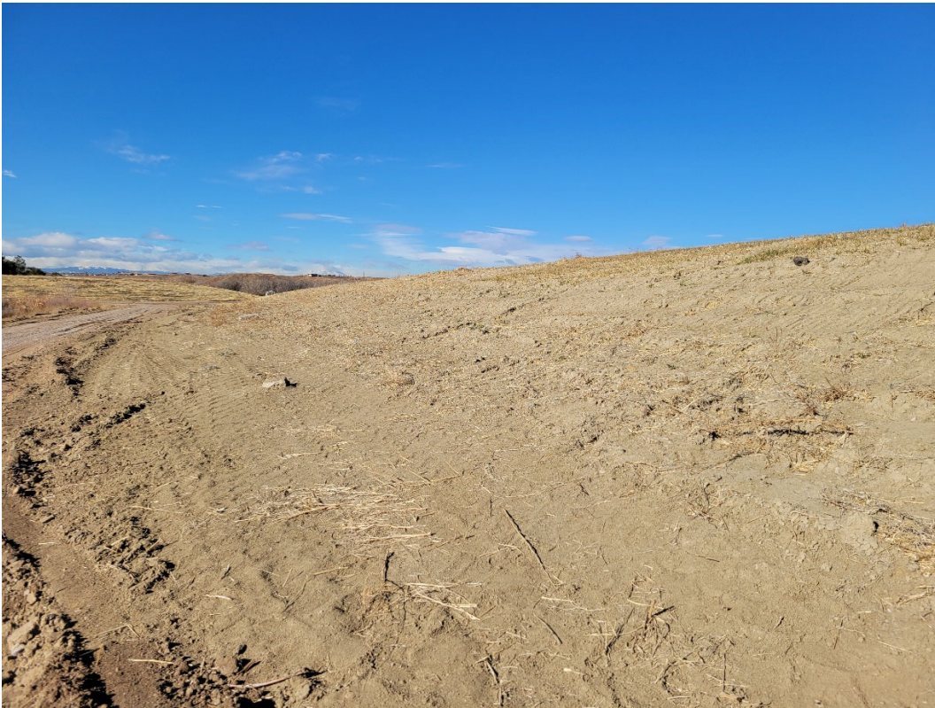
Photo 11: Side slope along the access road on the north end of the permit area. This area has not been seeded or mulched.
