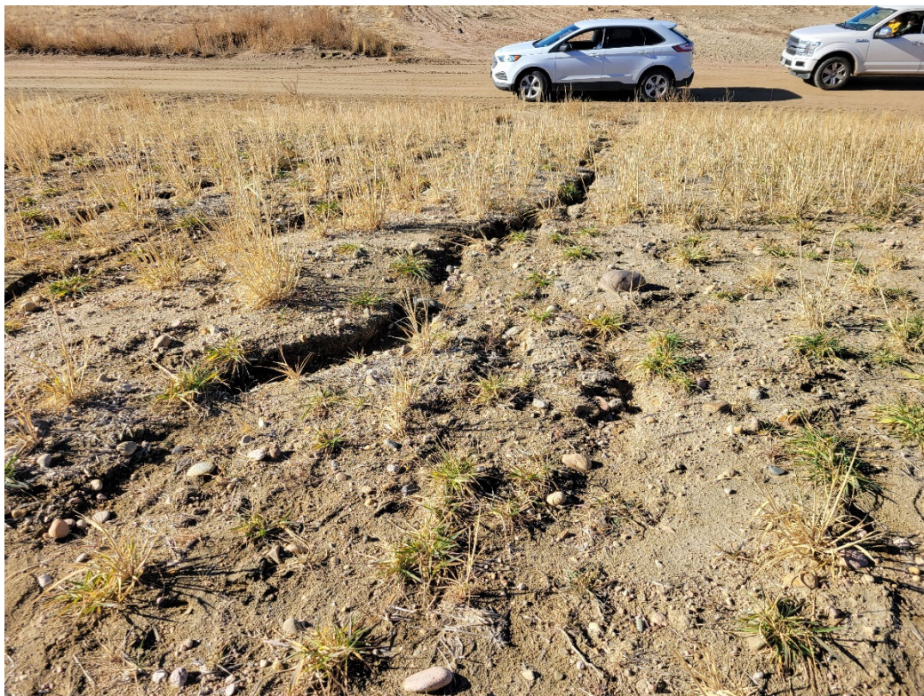
Photo 12: Erosion gullies observed on the western slope of the reseeded area near the entrance, on the south end.
