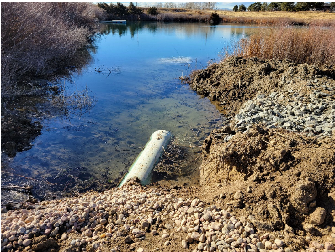
Photo 8: Discharge point for the French drain on the north end of the permit area.
