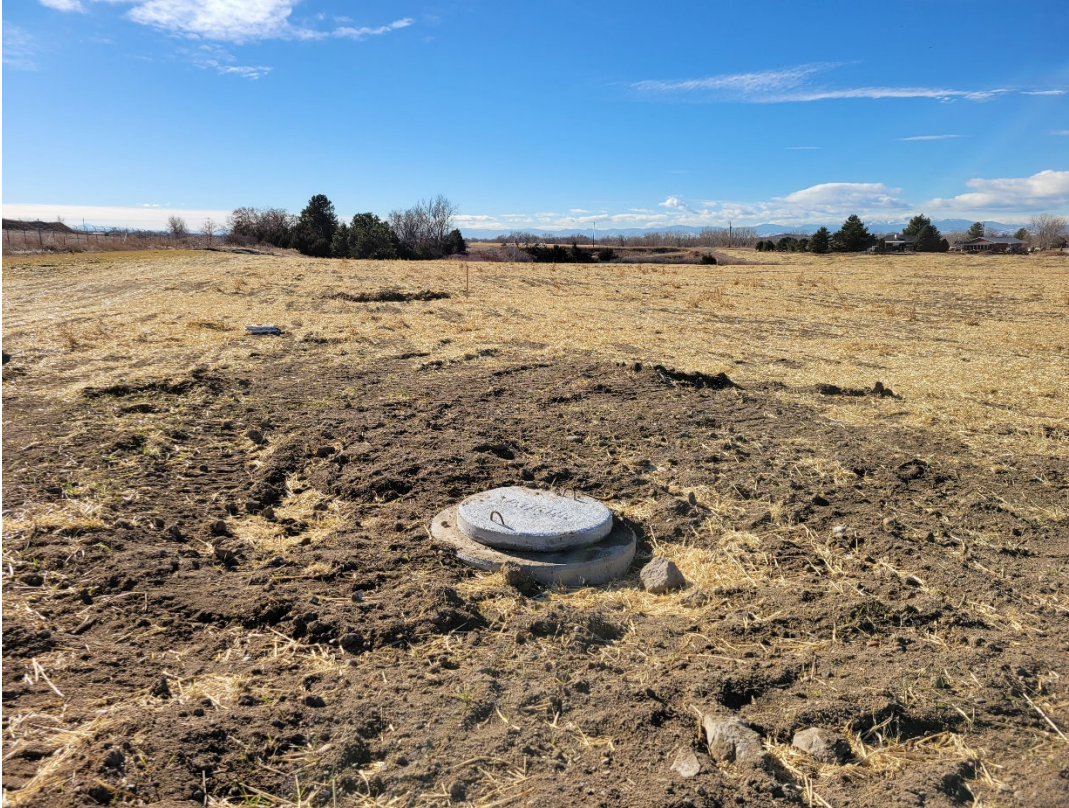
Photo 9: Manhole cover for the French drain along the eastern side of the clay lined inert fill area.
