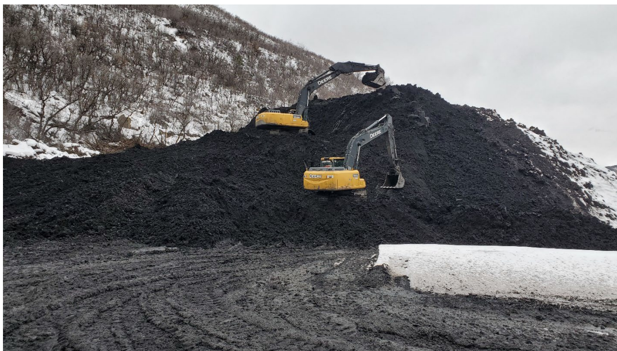
Figure 5: Two excavators used to raise height of temporarily piled waste on RPEE
