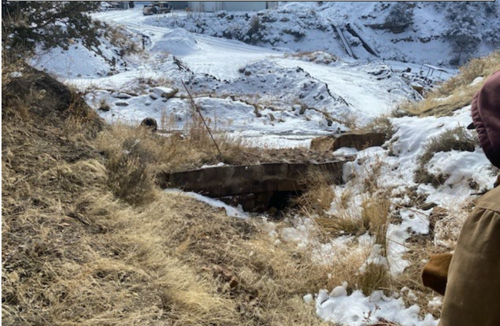
Photo 2: Maintenance Item No. 3, Sump B needs to be cleaned as soon as ground conditions will allow.
