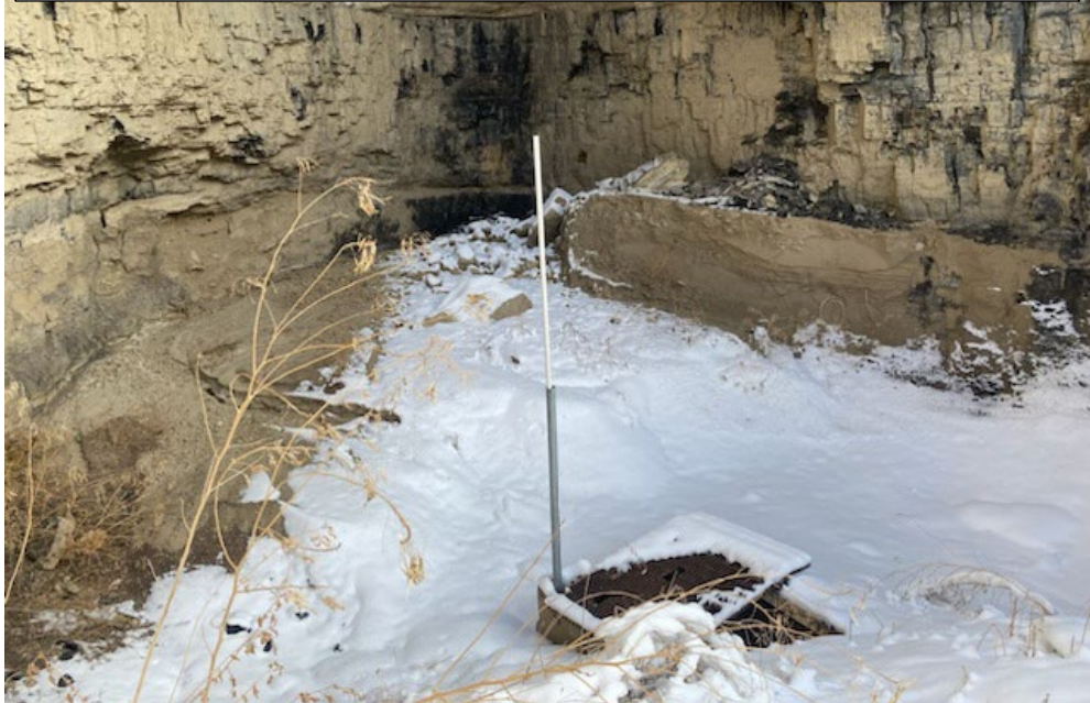
Photo 3: Maintenance Item No. 4, the trash rack on Sump D needs to be pulled all the way over the sumps outlet.
