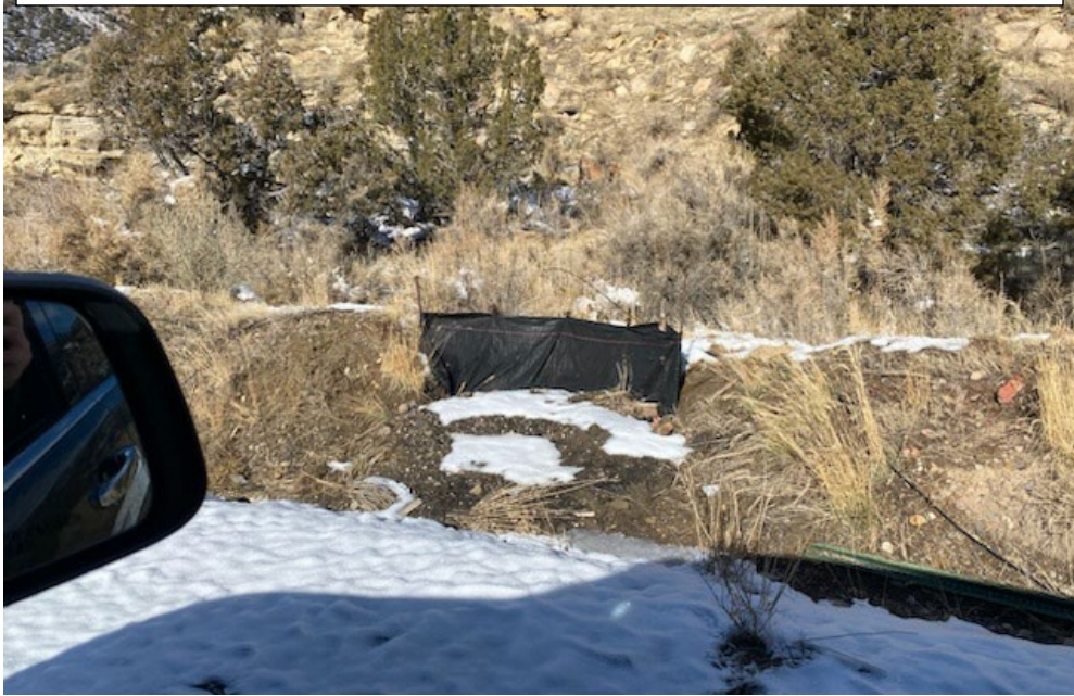
Photo 1: Maintenance Item No. 2, Sump P needs to be cleaned as soon as ground conditions will allow.
