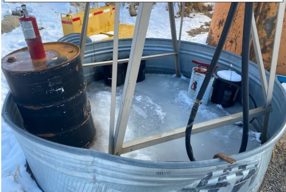
Photo 12: The secondary containment structure at the mine office pad.
