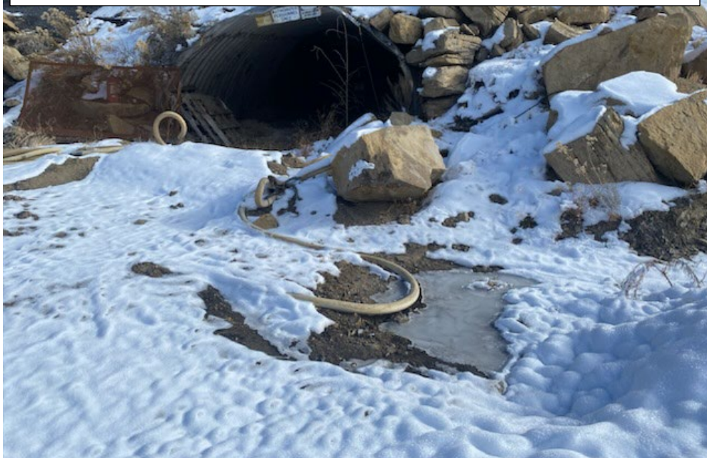
Photo 4: Maintenance Item No. 5, the cable laying on the ground in front of the portals need to be moved to a proper storage area.
