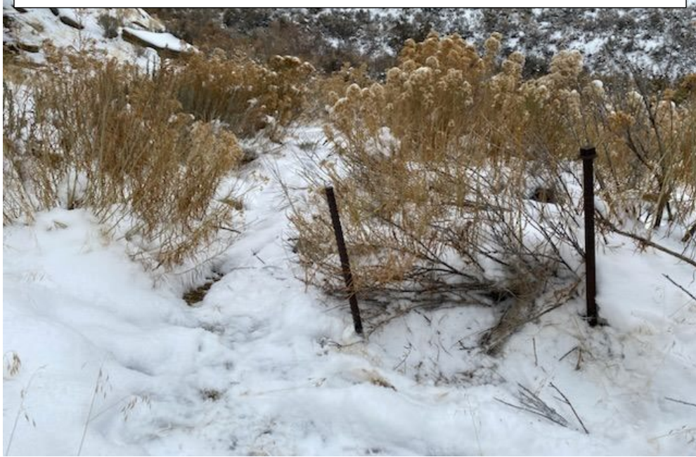
Photo 2: The Stakes at the Outlet Channel from the Explosives Storage Pad That Need to Have the Straw Bales Replaced.
