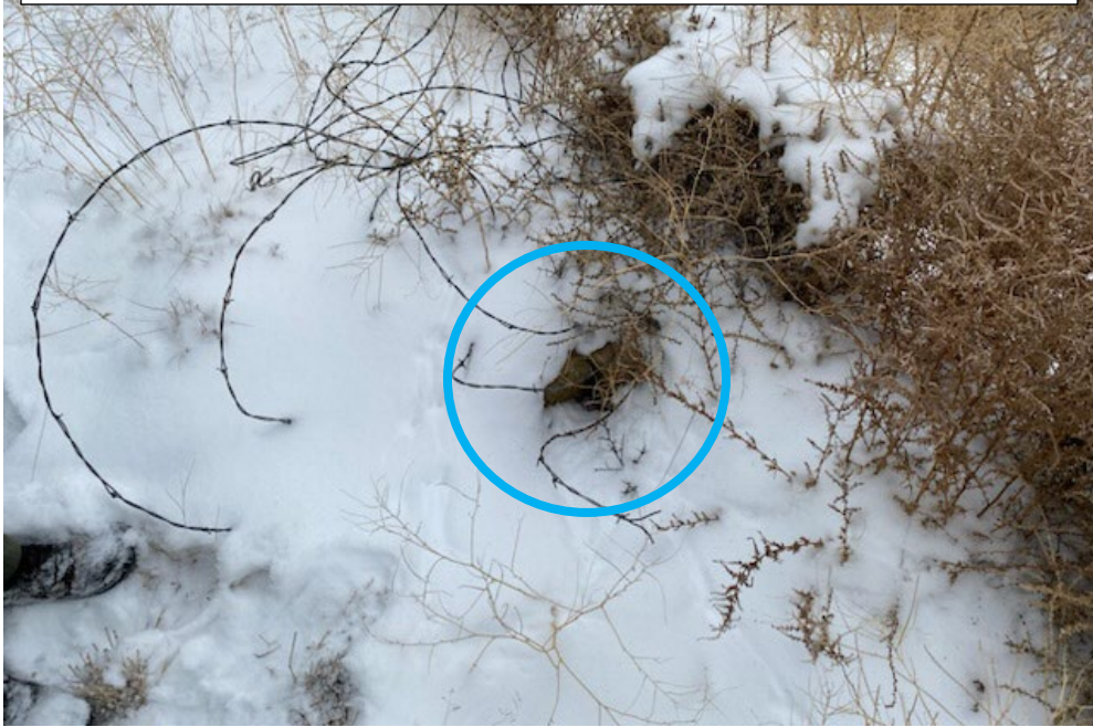
Photo 8: The Burrow Located on the Last Chance Pond's Embankment.
