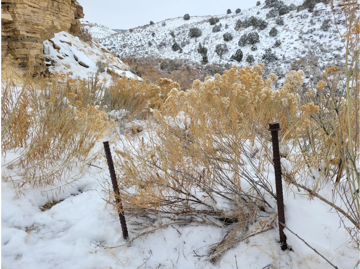
Figure 2. Explosives storage disturbed area runoff treatment; straw bale missing.
