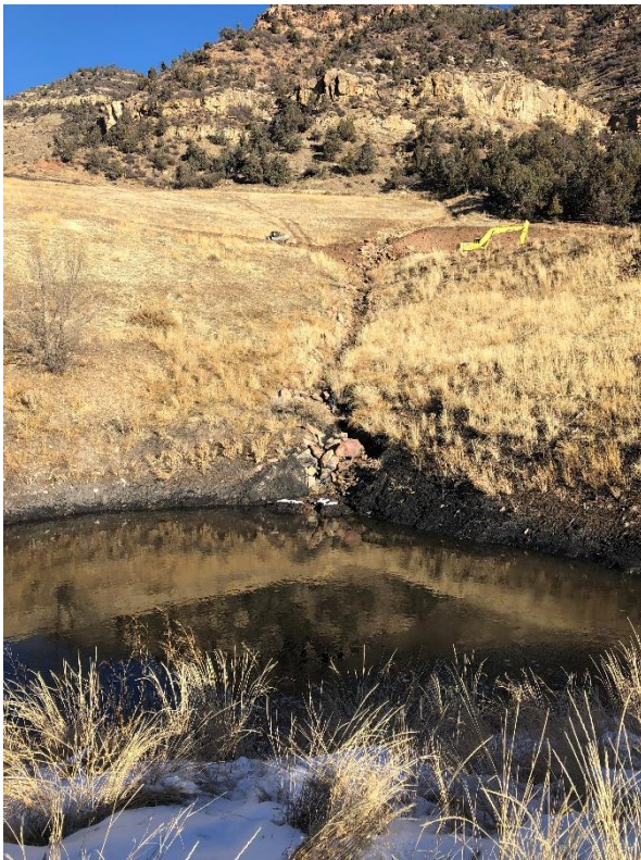
Erosion of inlet at Pond F
