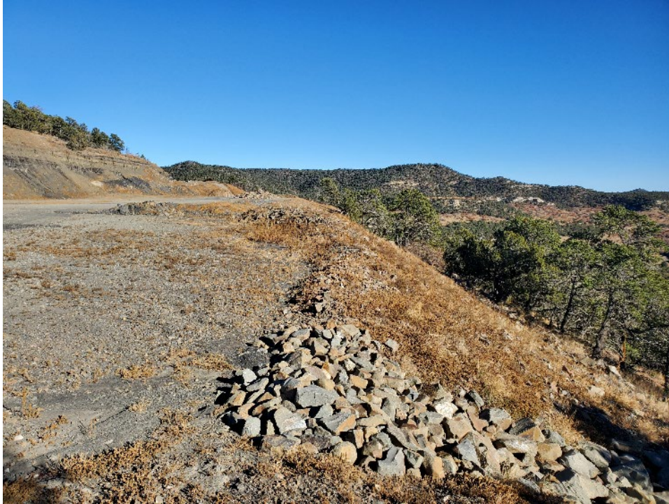
Photo 9: Looking east at an armored channel installed to help with sediment control onsite.
