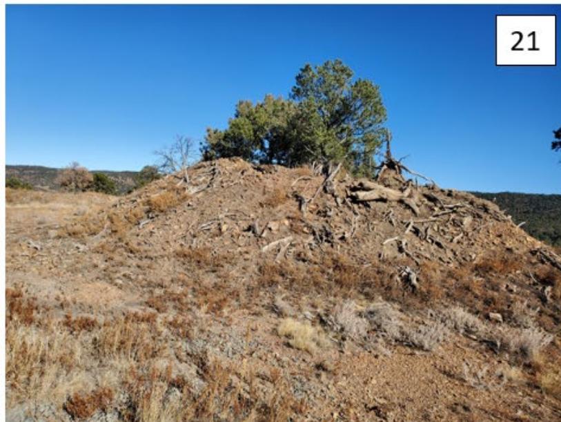
Photos 18-21: Photos 18-20 are topsoil piles that were marked with signs. Photo 21 shows a stockpile that the Operator stated is also topsoil. The piles in Photos 20 and 21 contain large woody material.
