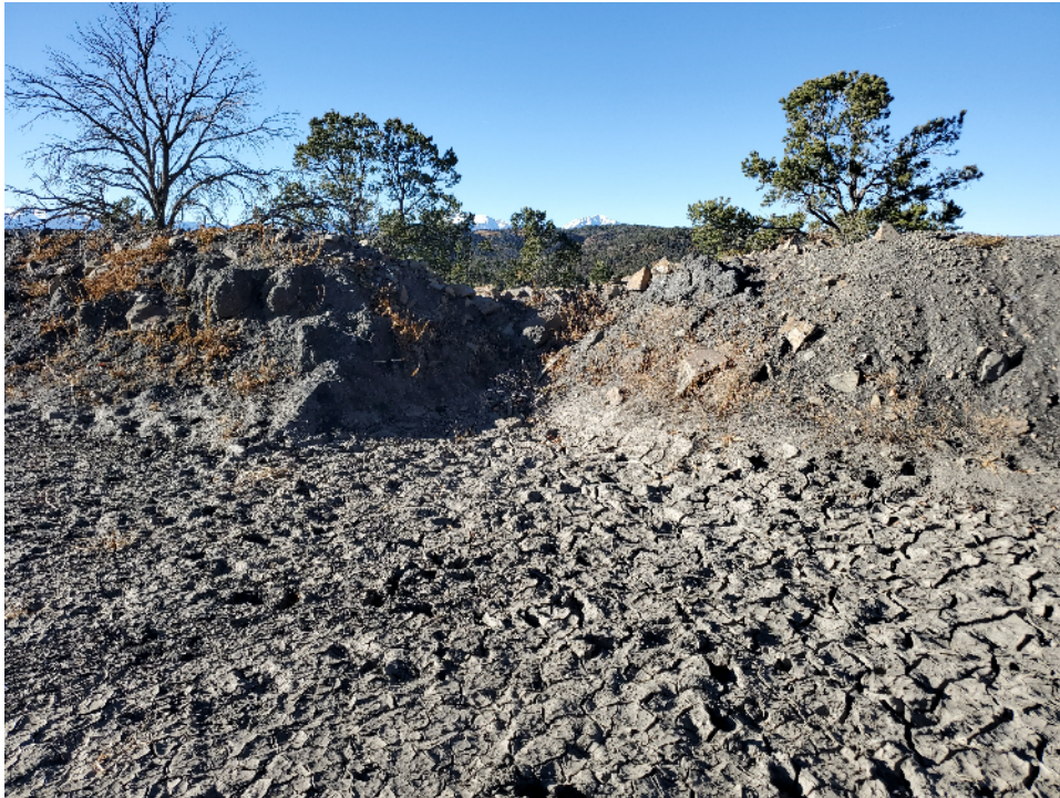
Photo 8: Looking west at an area along the pit boundary that had accumulated water. The berms in place have helped to control sedimentation and erosion from leaving the site in this area.
