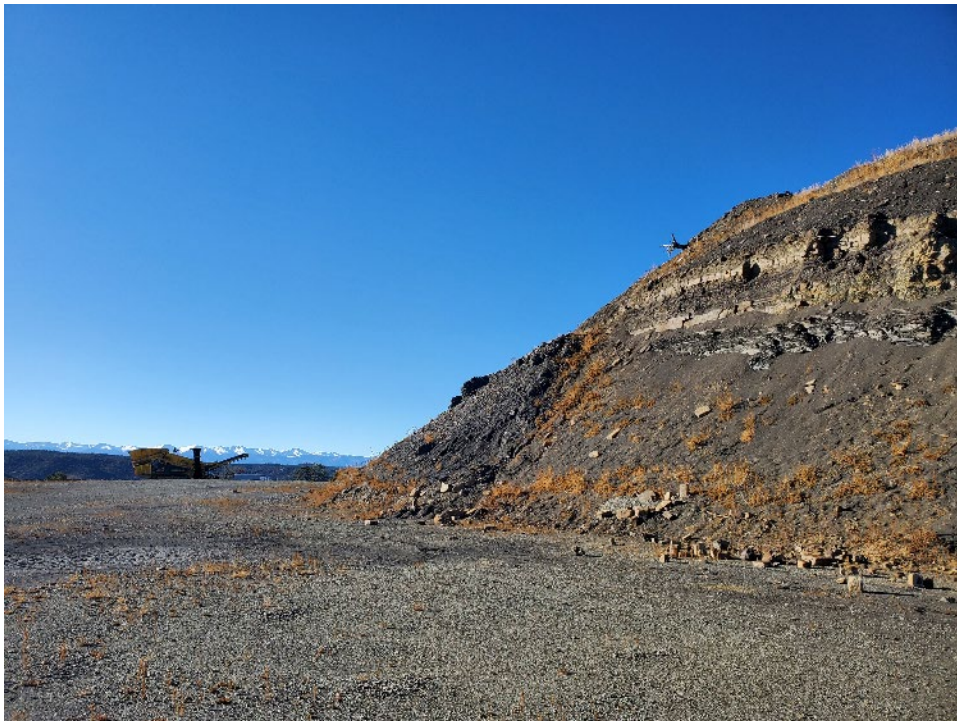
Photo 6: Looking west along the highwall in the pit area. The maximum height of the highwall is estimated at 17' from field measurements.
