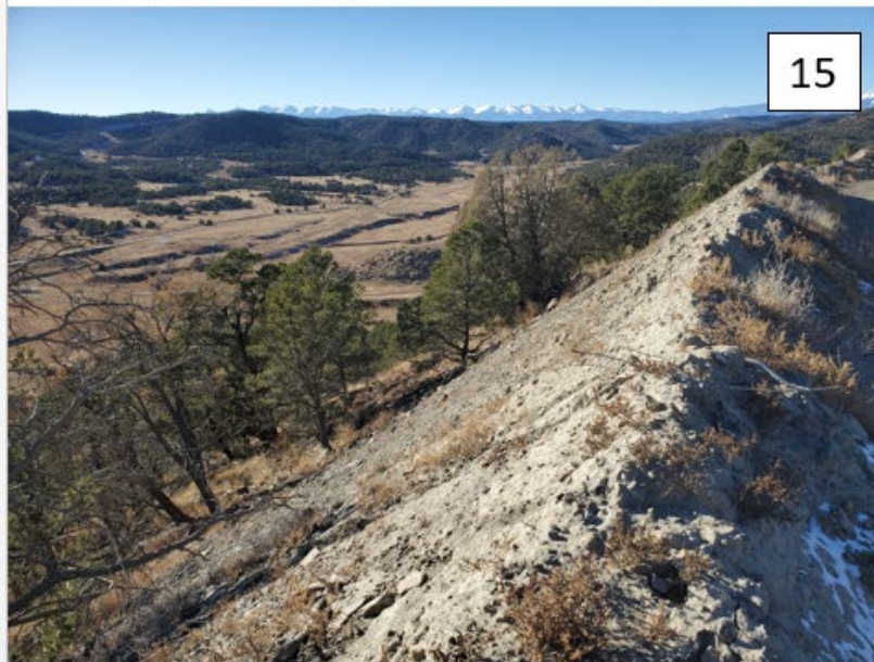
Photo 13-16: Photos 13 and 14 are looking downslope, and Photos 15 and 16 are looking across, the MSHA berms in the south-west portion of the permit. Sliding has occurred downslope of these berms.
