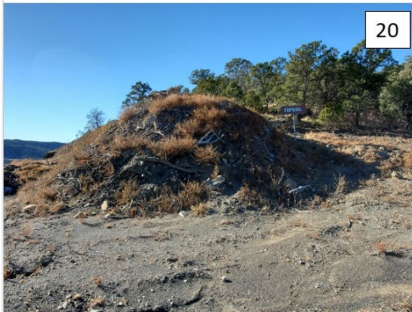
Photos 18-21: Photos 18-20 are topsoil piles that were marked with signs. Photo 21 shows a stockpile that the Operator stated is also topsoil. The piles in Photos 20 and 21 contain large woody material.
