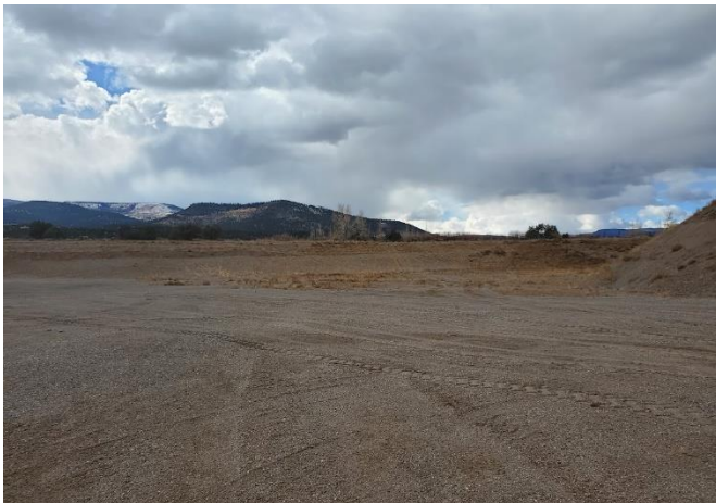
View to the southwest of southwest corner of the pit. Pit walls are at reclamation grade. No signs of exposed groundwater.
