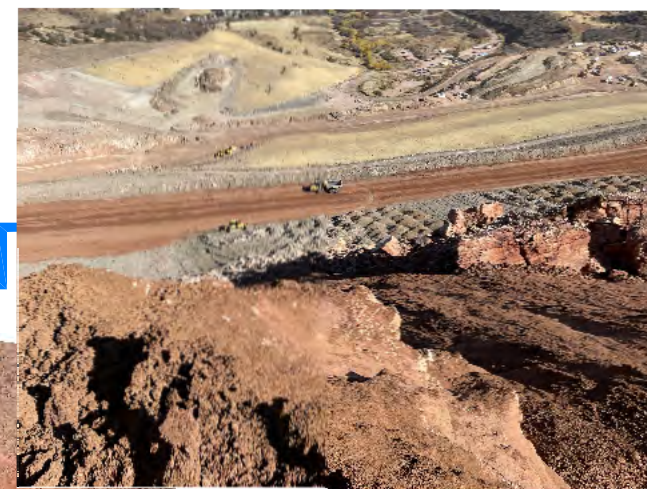
4. Material placed on bench for compaction.
