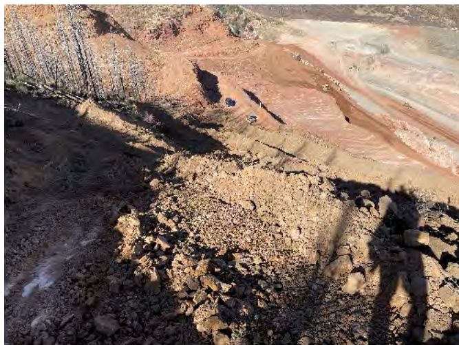
6. Access road pioneered to top of slope cut.
