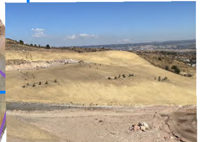
2. Graded borrow area with growth medium.
