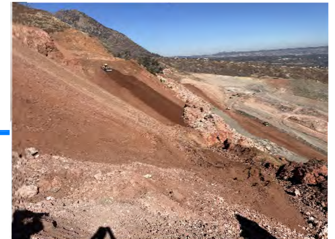
3. Dozer pushing material down from Upper Borrow Area to create access to Buttress.
