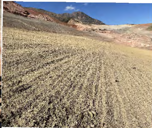
5. Slope below first bench. Hydroseeded and mulched
