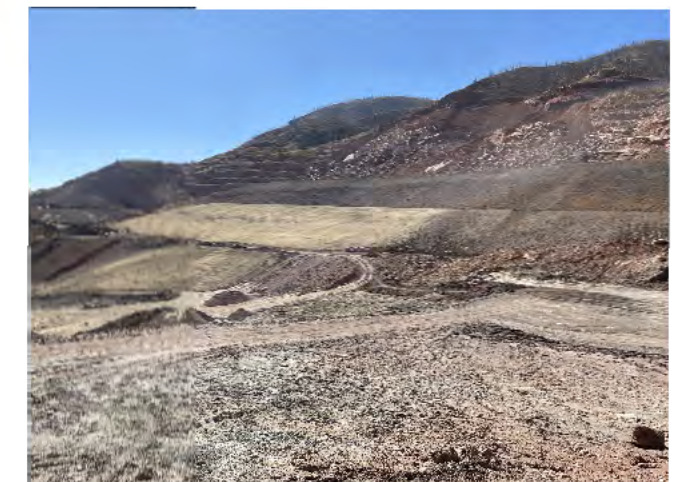
1. Bench slope at final grade.
