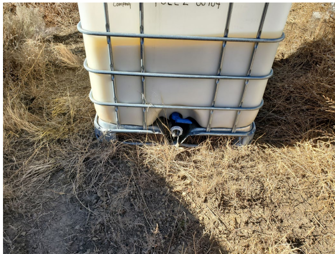
Photo 13: Single tank with noticeable leak.
