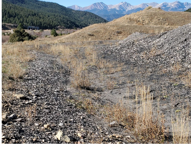
Photo 1: East side of the berm around D15 that needs to be raised.
