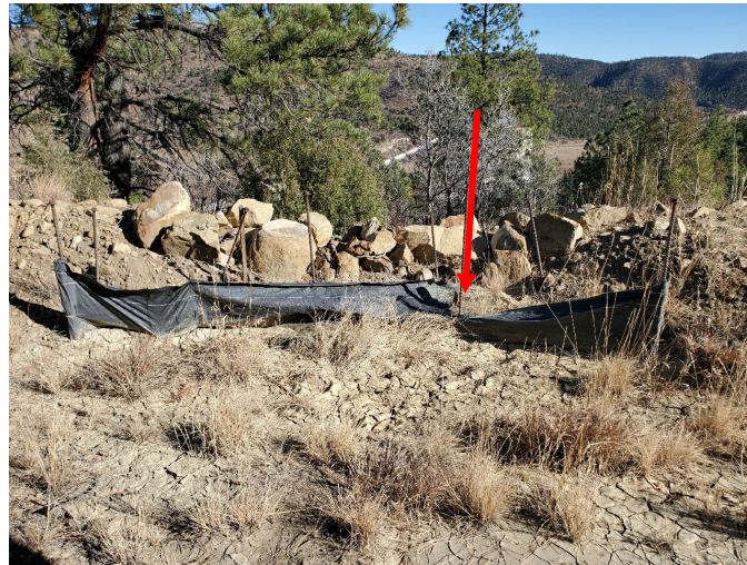
Photo 5: Damaged silt fence on western side of S.A.E.
