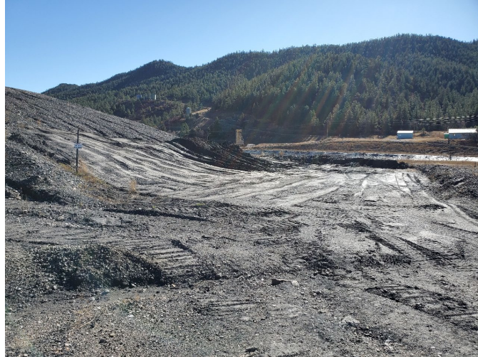
Photo 3: East side of DWDA #2 where ditch and pond cleanings are placed to dry.
