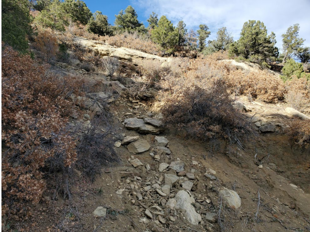
Photos 8A & 8B: Areas along D55 that are exhibiting failure. 8A – Slide up-slope of D55. 8B – Slide down-slope of D55.
