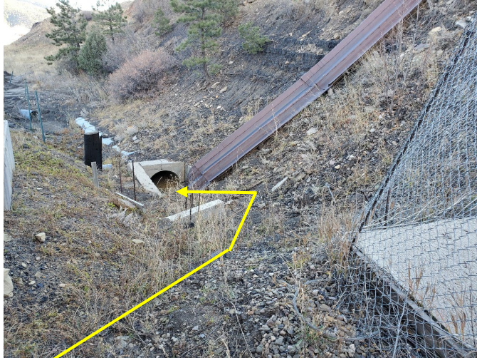
Photo 6: Arrow indicates water direction of water flowing south of the Fan, into the base of the Clean Water Flume, and into C48.
