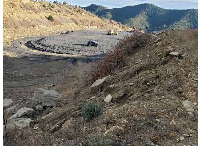
Photos 8A & 8B: Areas along D55 that are exhibiting failure. 8A – Slide up-slope of D55. 8B – Slide down-slope of D55.
