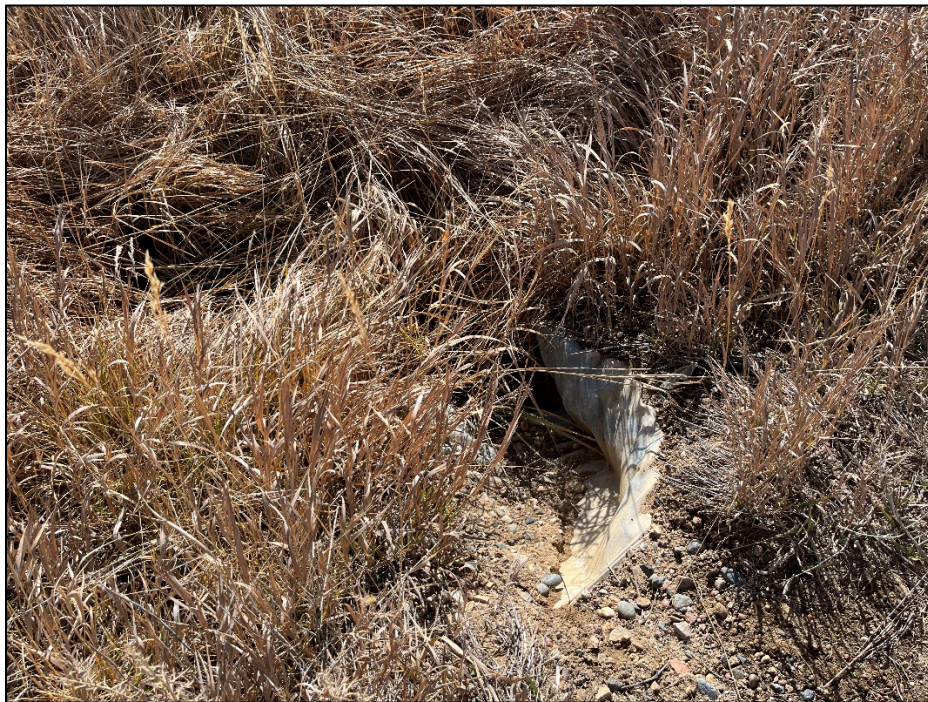
Photo 12: Crushed culvert at the southern end of the NPDES #7 discharge point, in need of repair.
