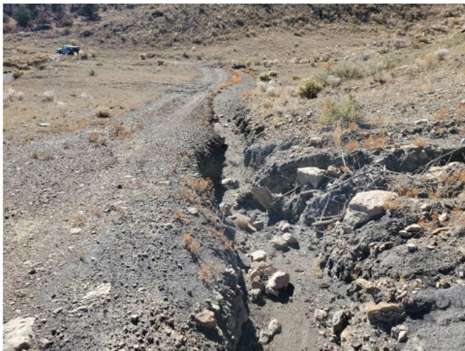
Photo 2: Erosion along south-east side of the reclaimed area above Pond 006a and along the road that's located between this area and Pond 006a.
