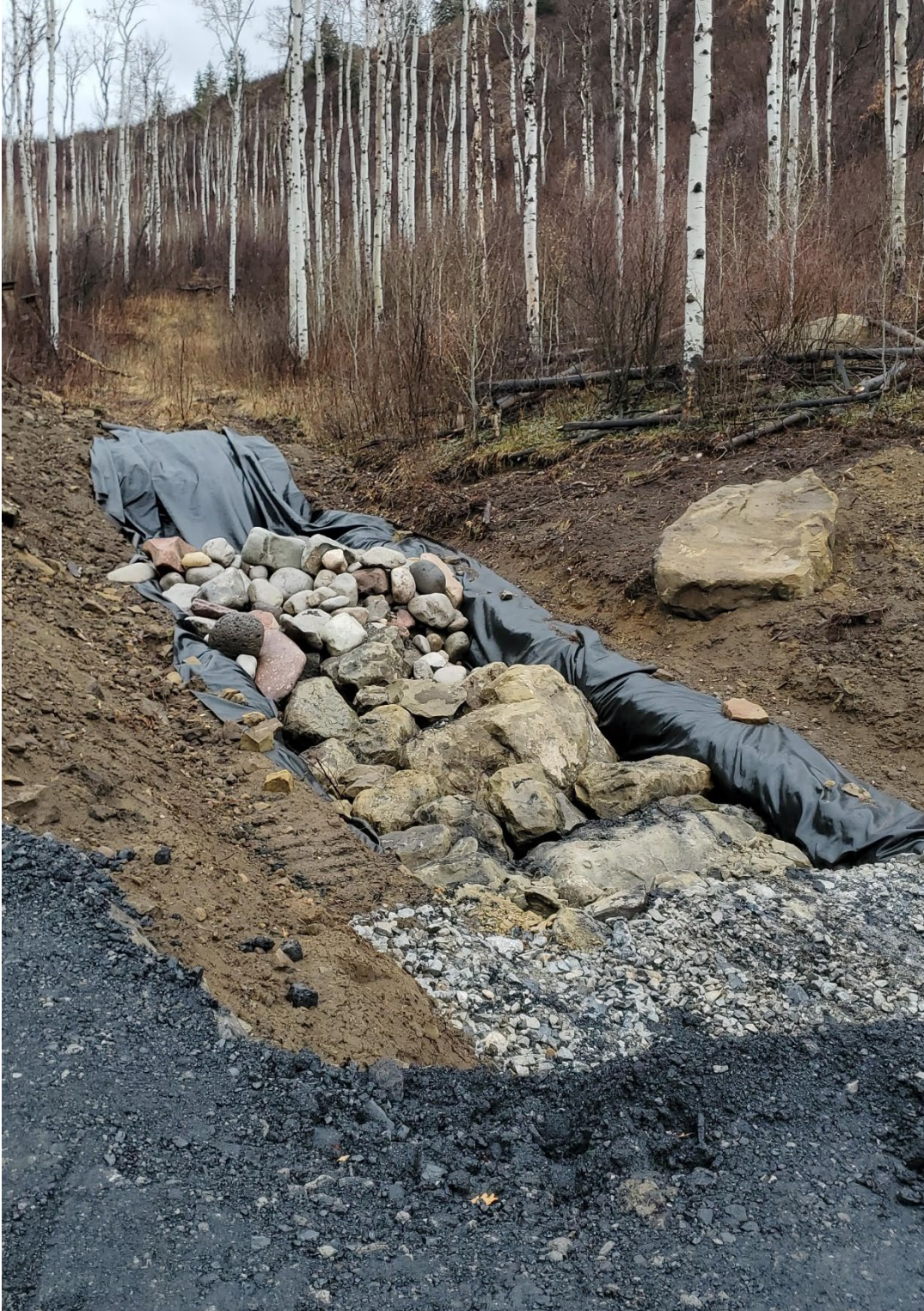
Figure 9: Underdrain on RPE
