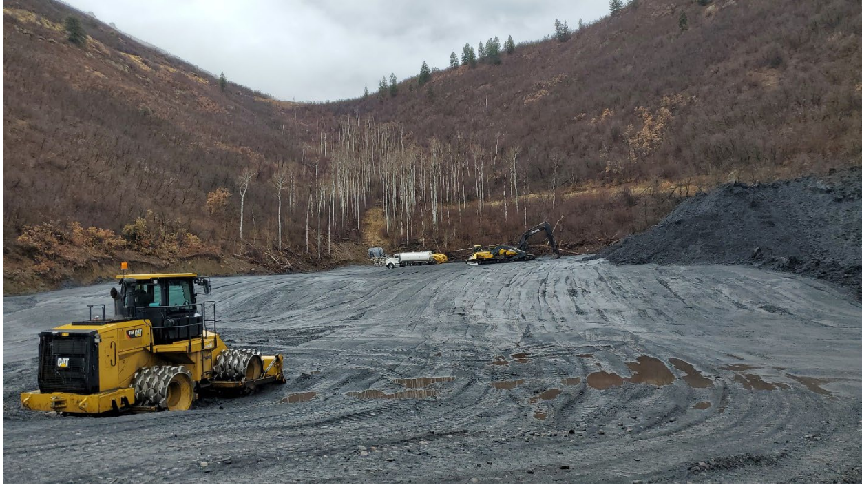
Figure 6: Compacted surface of RPEE, with uncompacted material on west side
