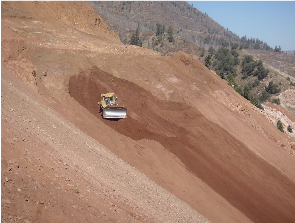
Photo 2. D9 dozer constructing upper access road (looking north).
