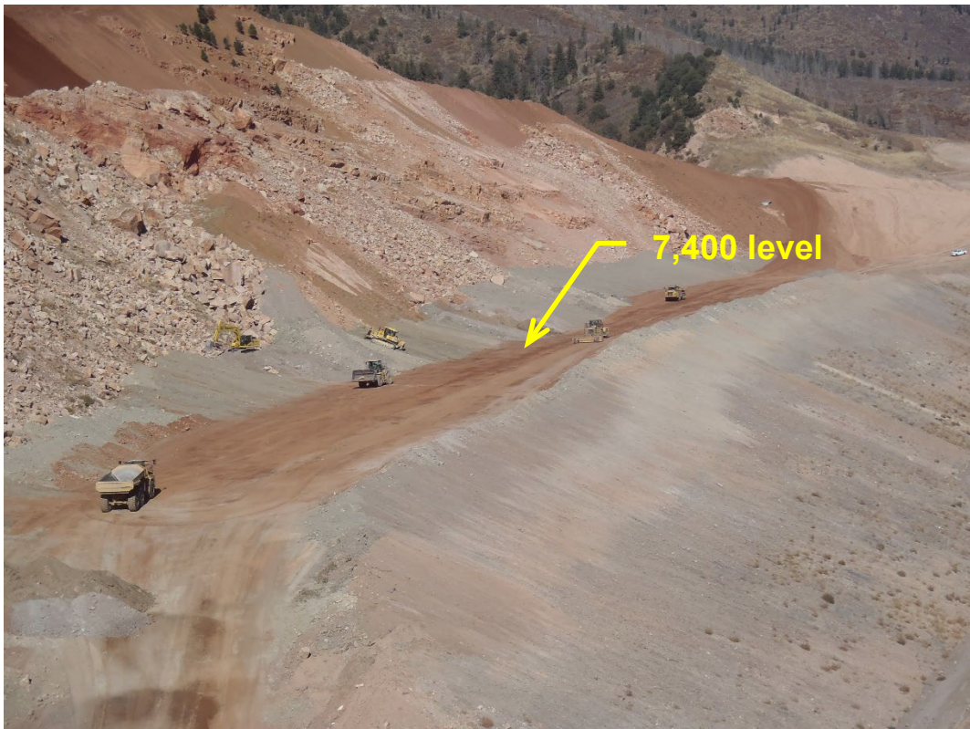
Photo 1. Buttress backfill at ~7400 foot level (looking north).
