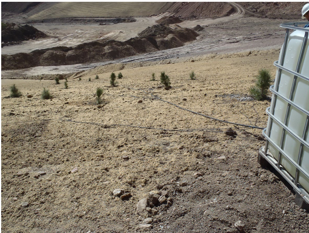
Photo 6. Newly planted conifers and typical irrigation system (former shop area).
