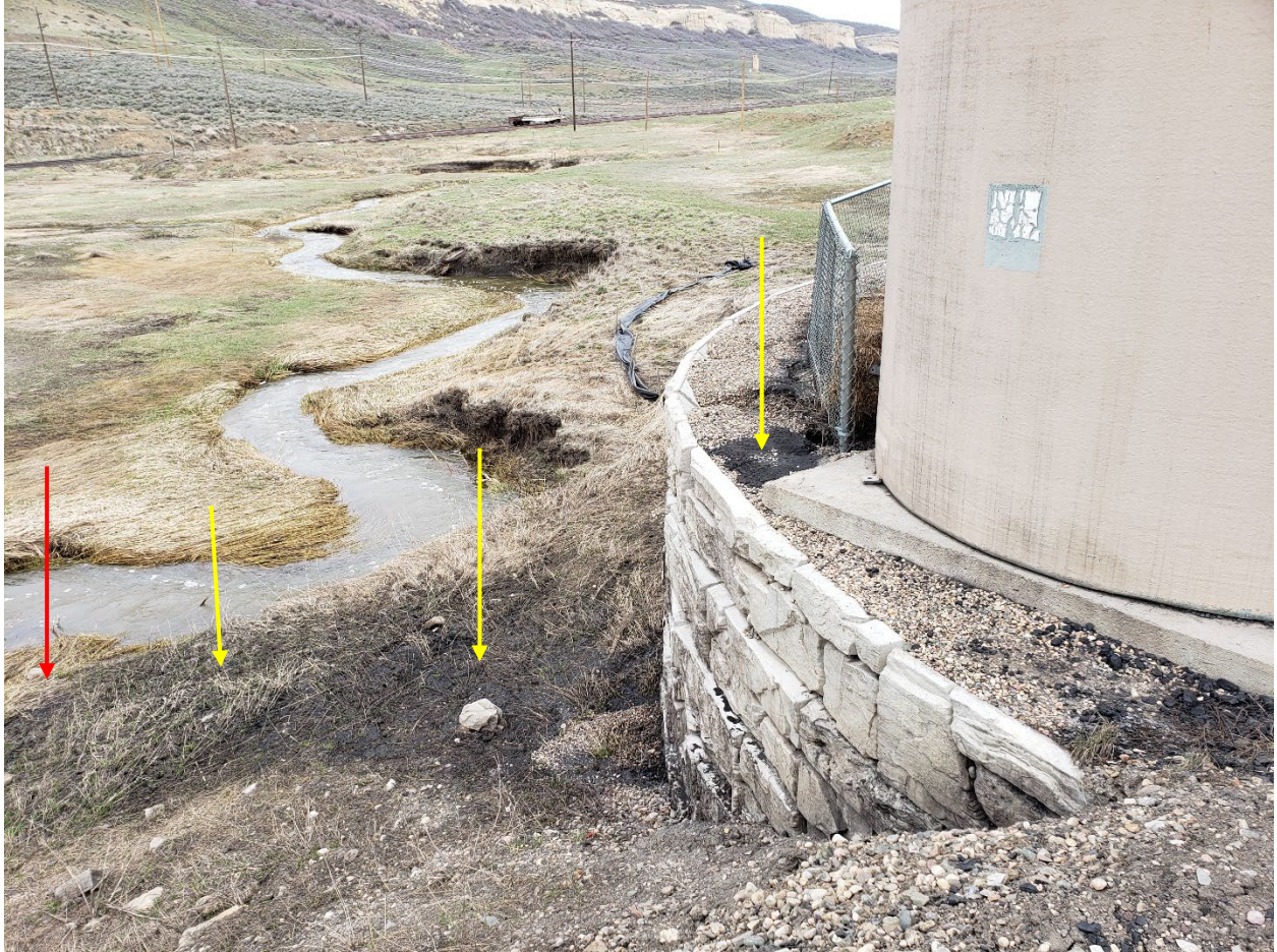
Figure 4 - An area of the stoker coal loadout that suggests flow is still escaping the sediment control system. Coal fines located beyond the hay bales at a location of significant erosion behind the retaining wall (yellow arrows) are also not currently sequestered behind any sediment control (red arrow).
