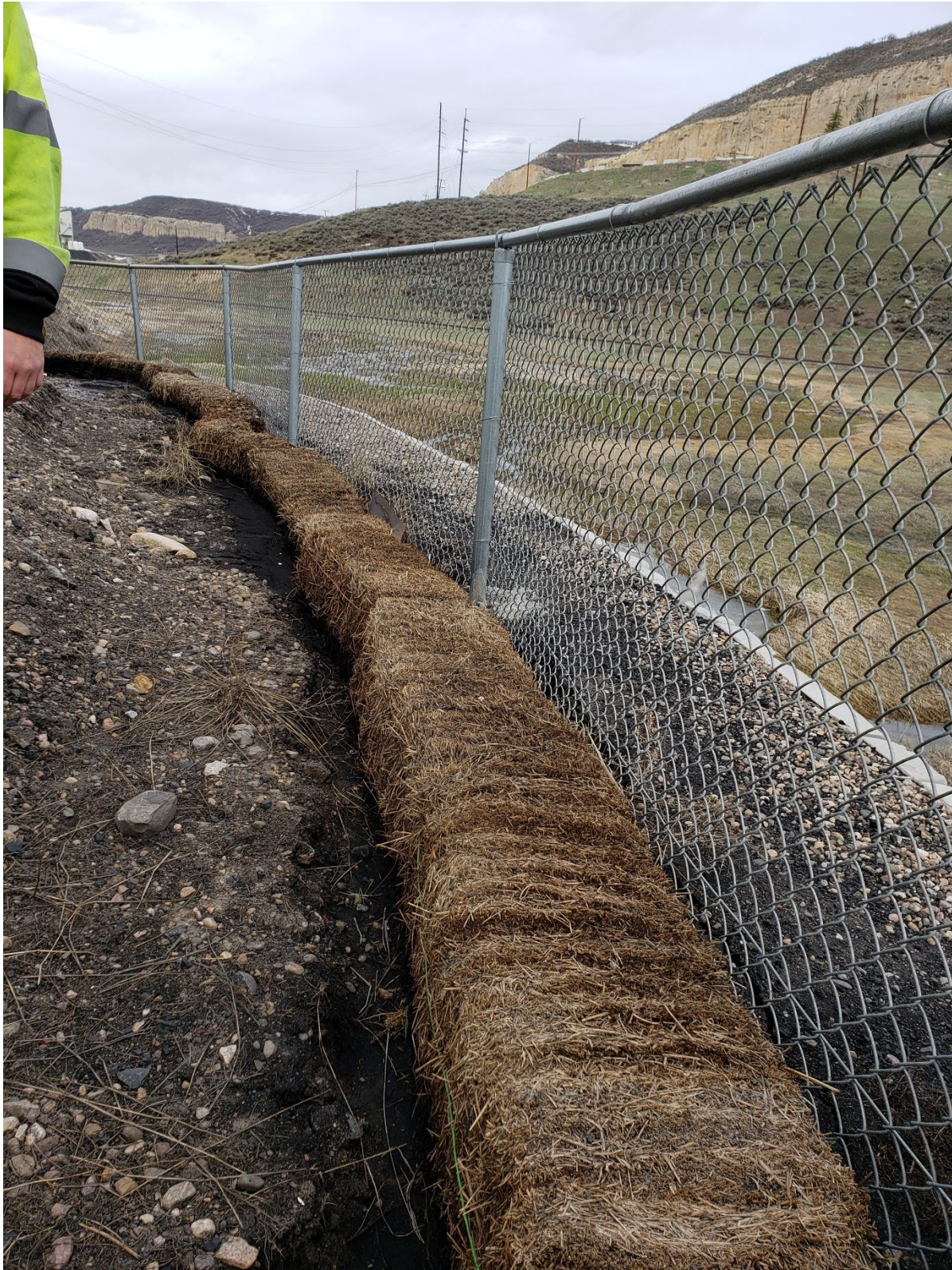
Figure 2 - Hay bales providing temporary protection against sediment from the stoker coal loadout flowing into the Foidel Creek drainage.
