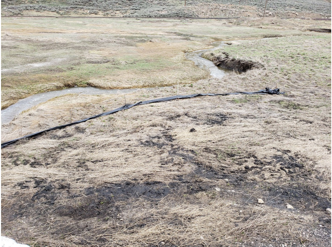
Figure 3 - Silt fence installed to prevent sediment from the stoker coal loadout from reaching Foidel Creek. This fence is in need of repair or removal, and the sediment requires removal.
