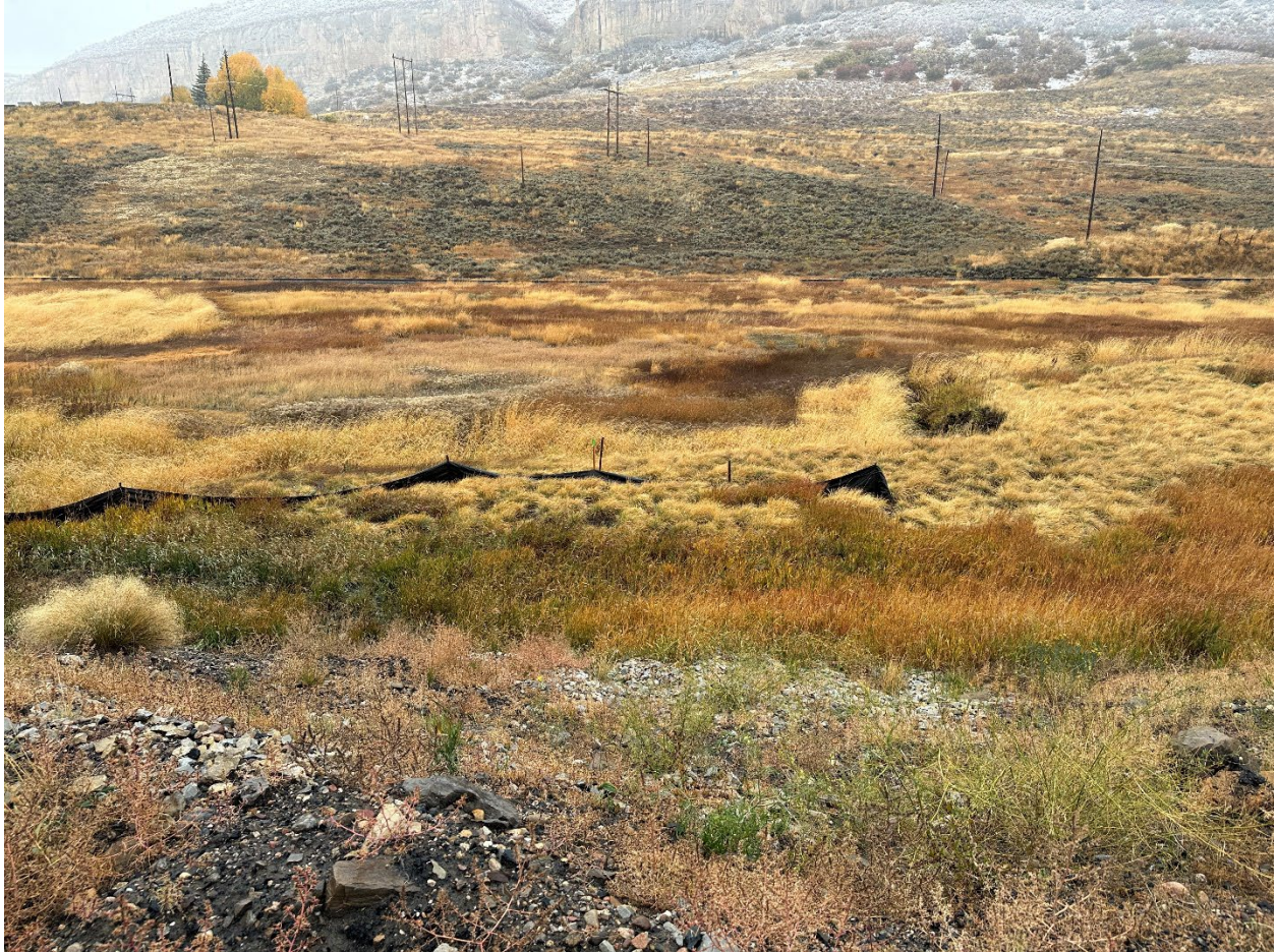
Figure 2 - The silt fence outside the Stoker Coal Loadout requires repair as the silt fence has slumped and become detached from several supporting posts.
