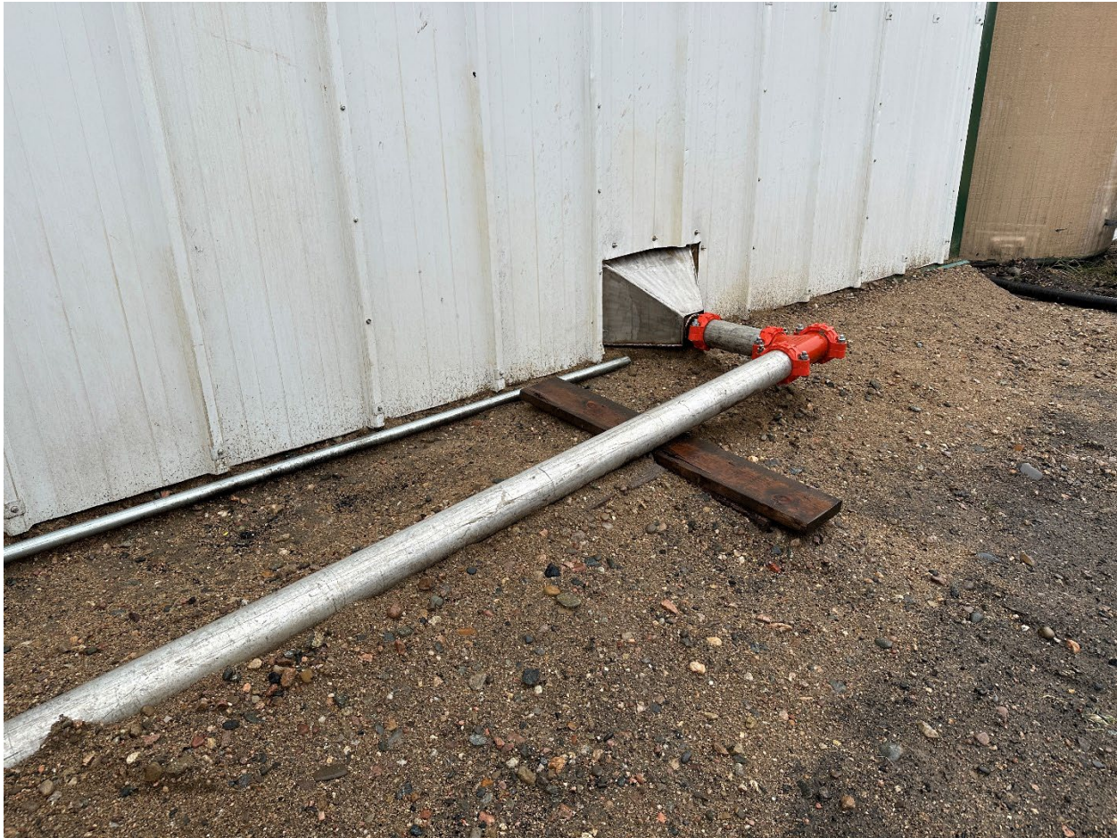
Figure 1 – The recently installed pipe directing water from the Stoker Coal Loadout to the pumphouse. The repair to prevent water and sediment from reaching Foidel Creek was fully functional at the time of inspection.
