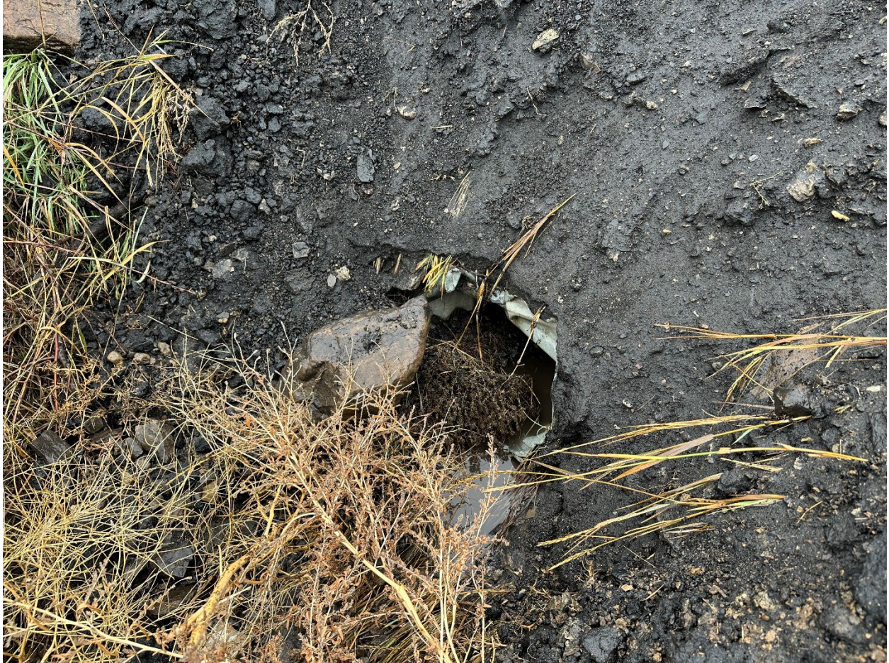
Figure 4 - A partially blocked culvert that requires clearing in the Pond E area.
