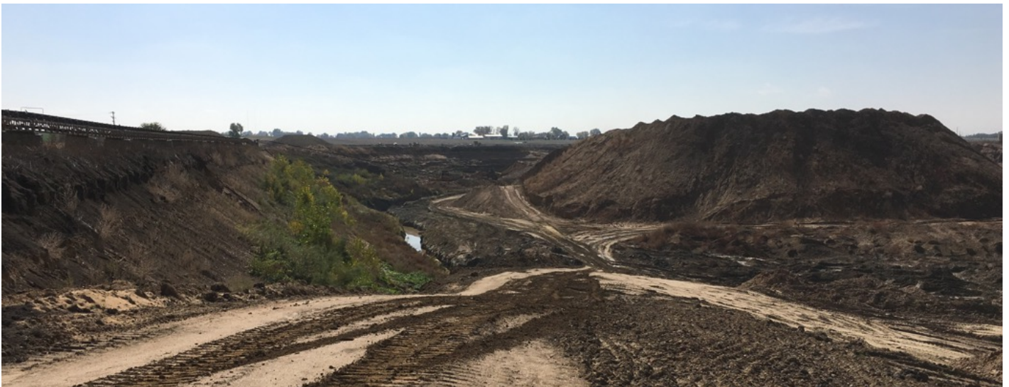
Figure 3 - Dewatering trench installed in shale bedrock during clay liner construction in October 2017.
