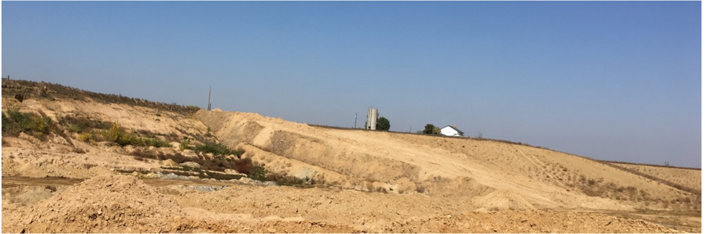
Figure 2 - Construction of clay liner in October 2017 along the western highwall of the gravel pit.
