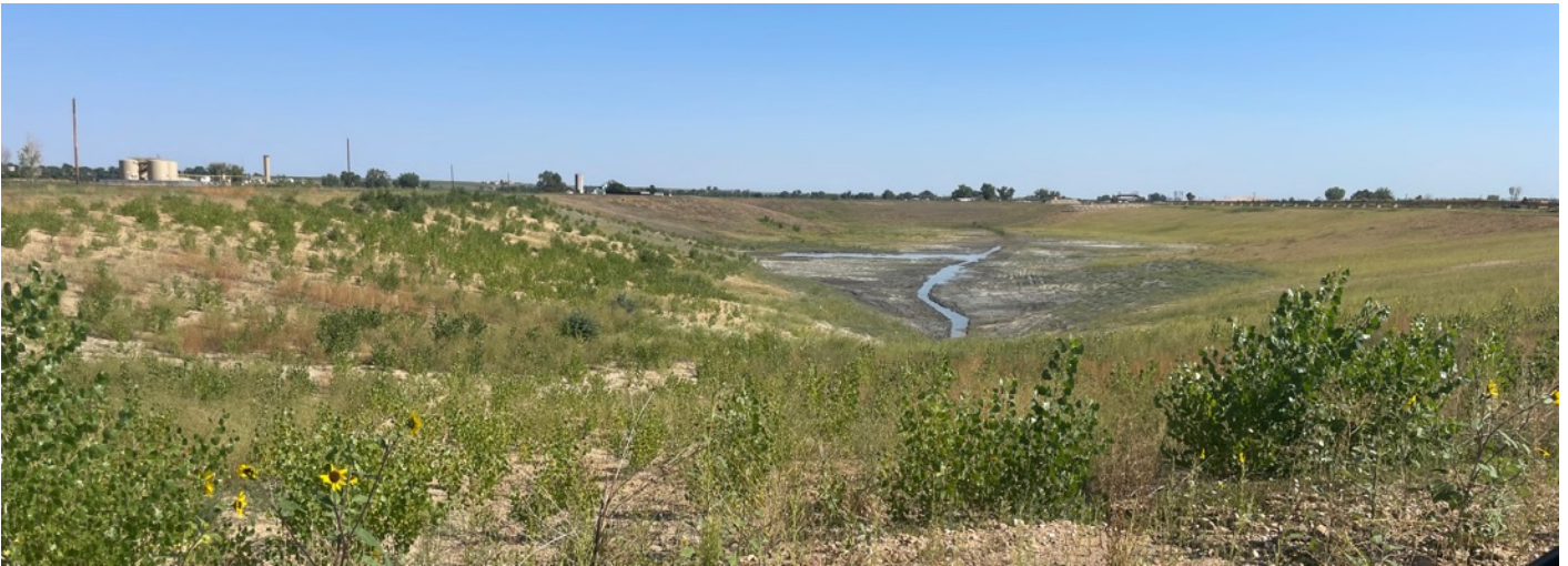
Figure 4 - Completed lined pit in August 2022 (view to the north).
