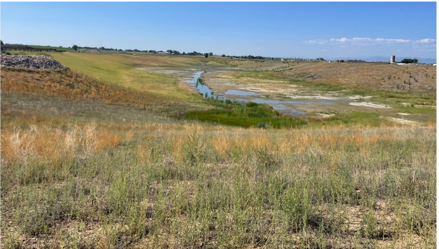
Figure 5 - Completed lined pit in August 2022 (view looking south) with wet well (far left side of photo).
